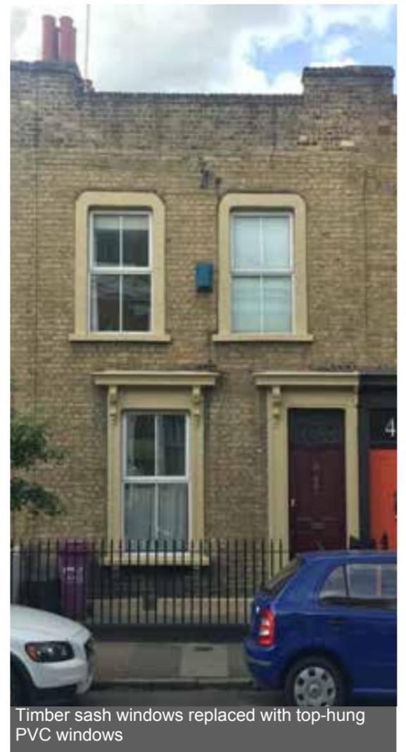
Timber sash windows replaced with top-hung PVC windows
