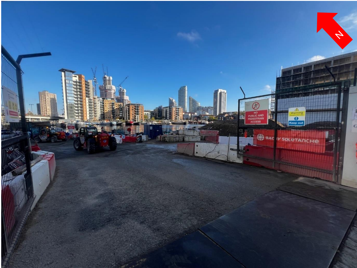
Figure 10: Image of the site in its current state from Brannan Street.
