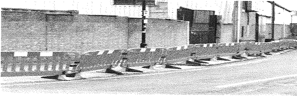
Fencing in Autumn Street erected after noise complaints
