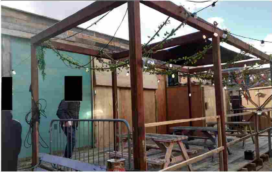
Image 8 - outs of the lounge area now enclosed
