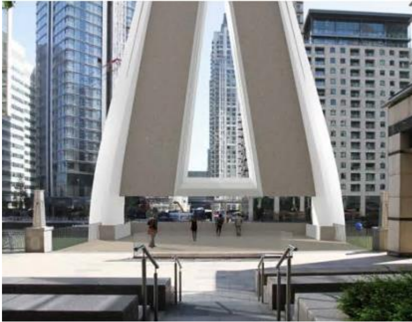
Figure 3: Bridge in 'open' position as seen from Upper Bank Street
