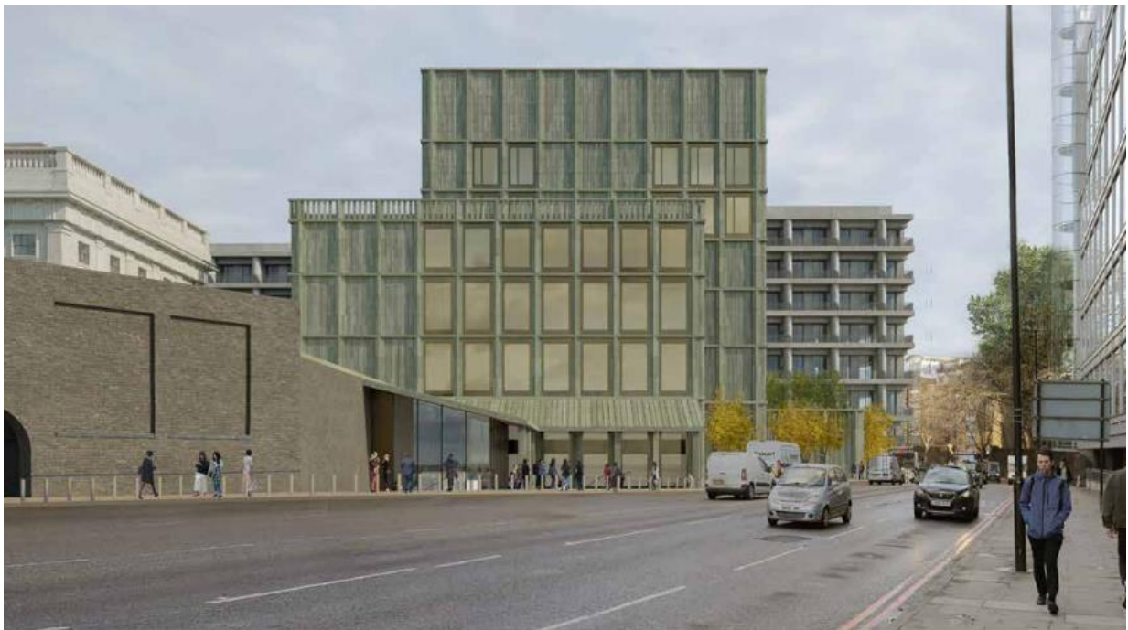
Figure 12: View of Cultural Exchange Building from East Smithfield
