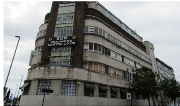
Fig. 15: Bow House Business Centre
