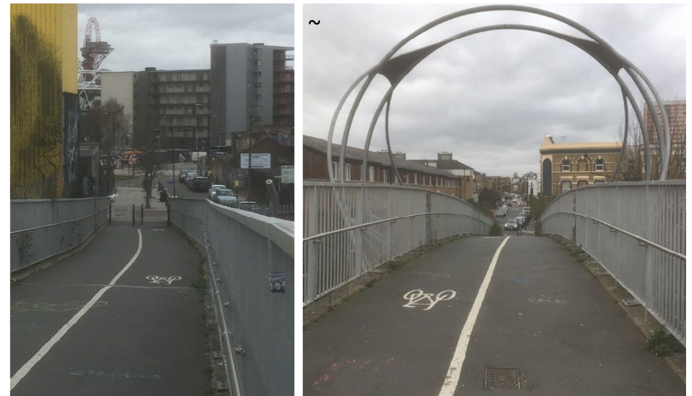
Fig. 8: Crown Close pedestrian bridge
