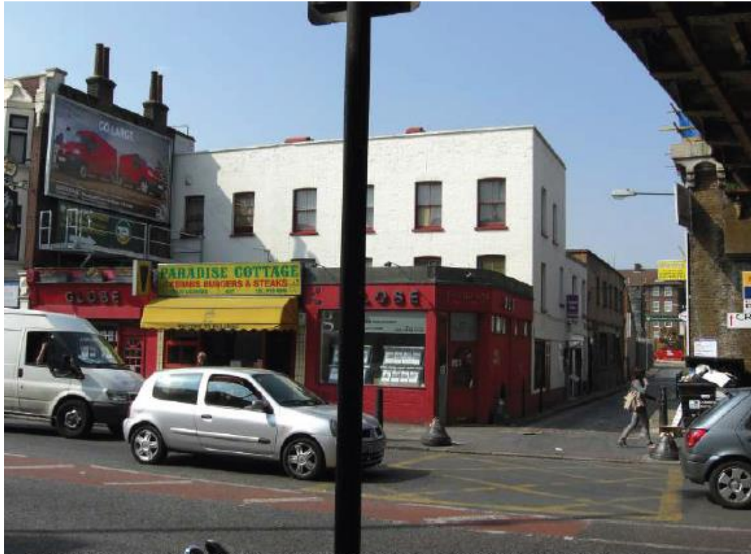
1 ENTRANCE TO HOLLYBUSH PLACE FROM BETHNAL GREEN ROAD
