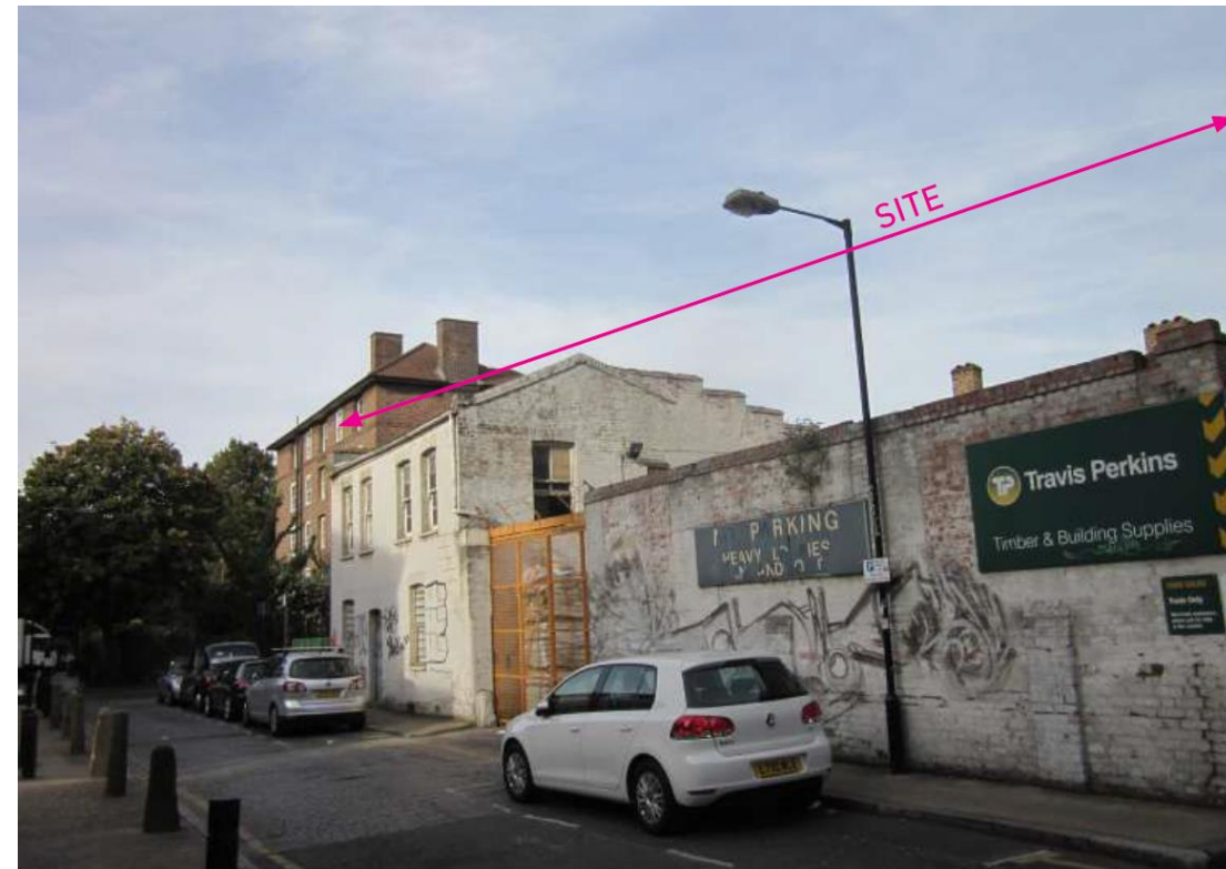
5 SITE FRONTAGE ALONG HOLLYBUSH GARDENS
