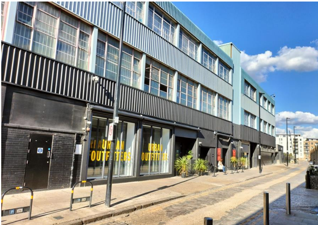
Appendix 2.3: View of photography/ filming studios entrance (nightclub at night) on Pennington Street
