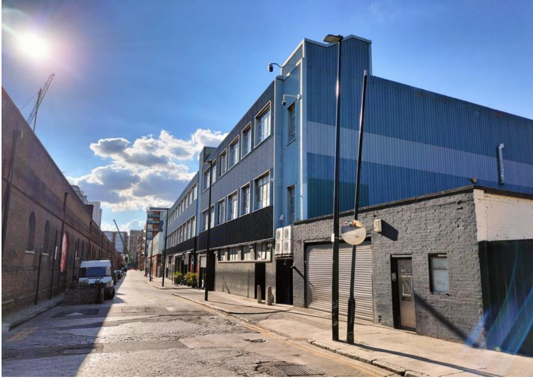
Appendix 2.2: View from east on Pennington Street towards photography and filming studios/ nightclub with self-storage above
