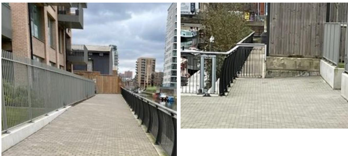
Figure 3: (Left to right) Eastern end of canal path blocked and western end of canal path blocked
