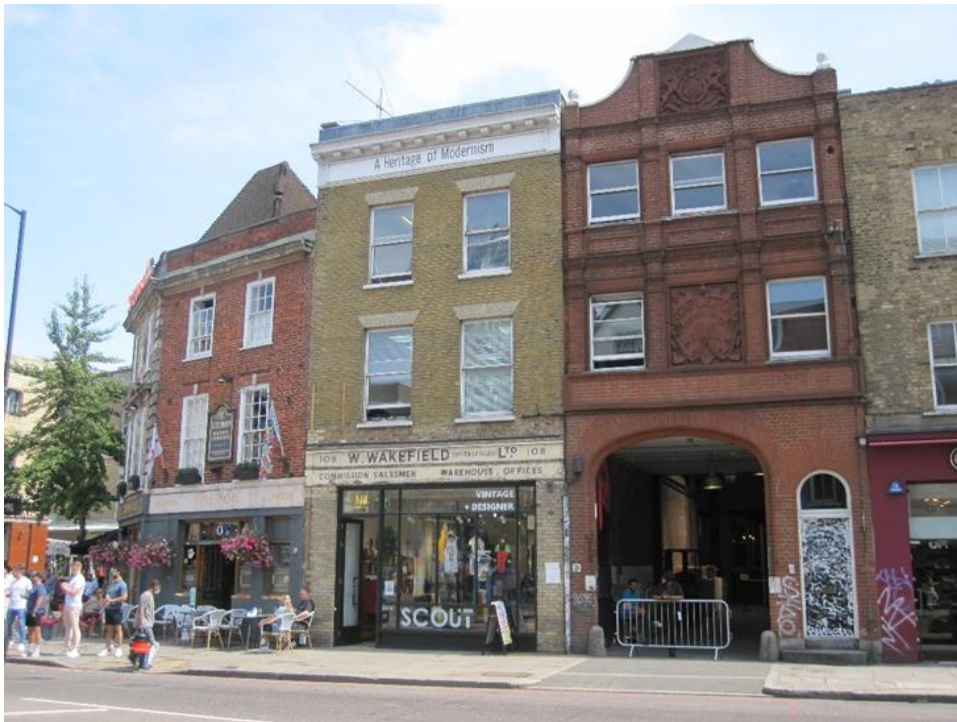
Existing view looking eastwards towards the main Commercial Street entrance
