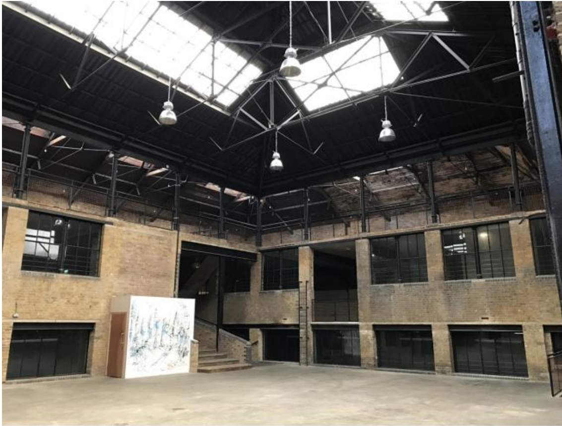
Figure 4: Interior view from ground floor looking towards the south east corner
