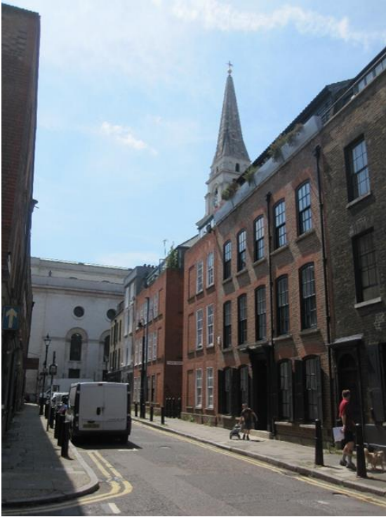
Existing view looking southwards along Wilkes Street (site is not visible)
