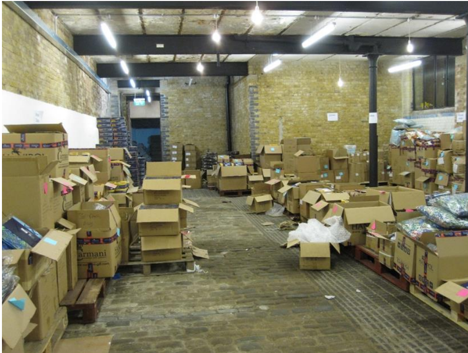
Interior view of existing basement with cobbled flooring visible
