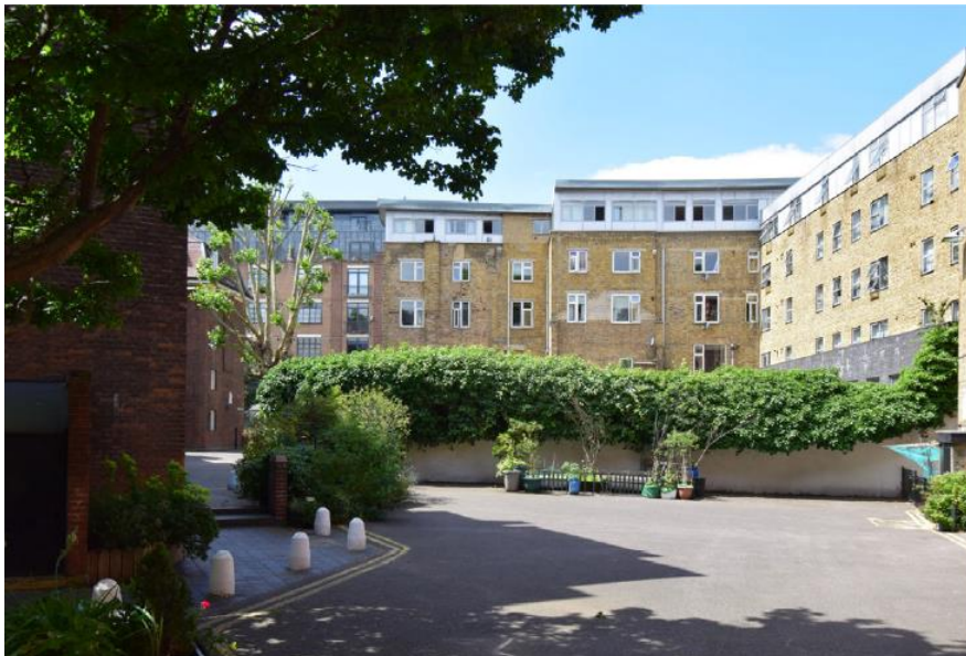
Figure 11: Existing view from Shiplake House Courtyard
