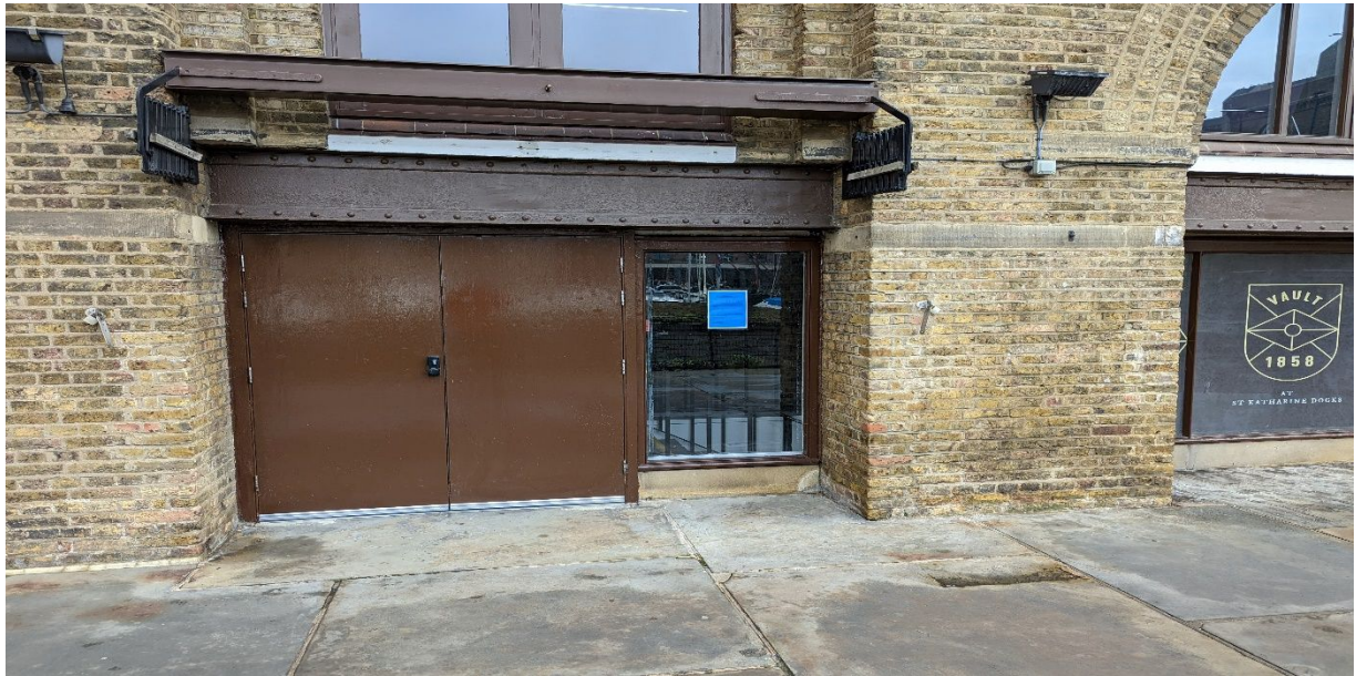
Images of the Premises – Dockside Vaults Ivory House St Katherine's Dock East Smithfield London E1W 1BP
