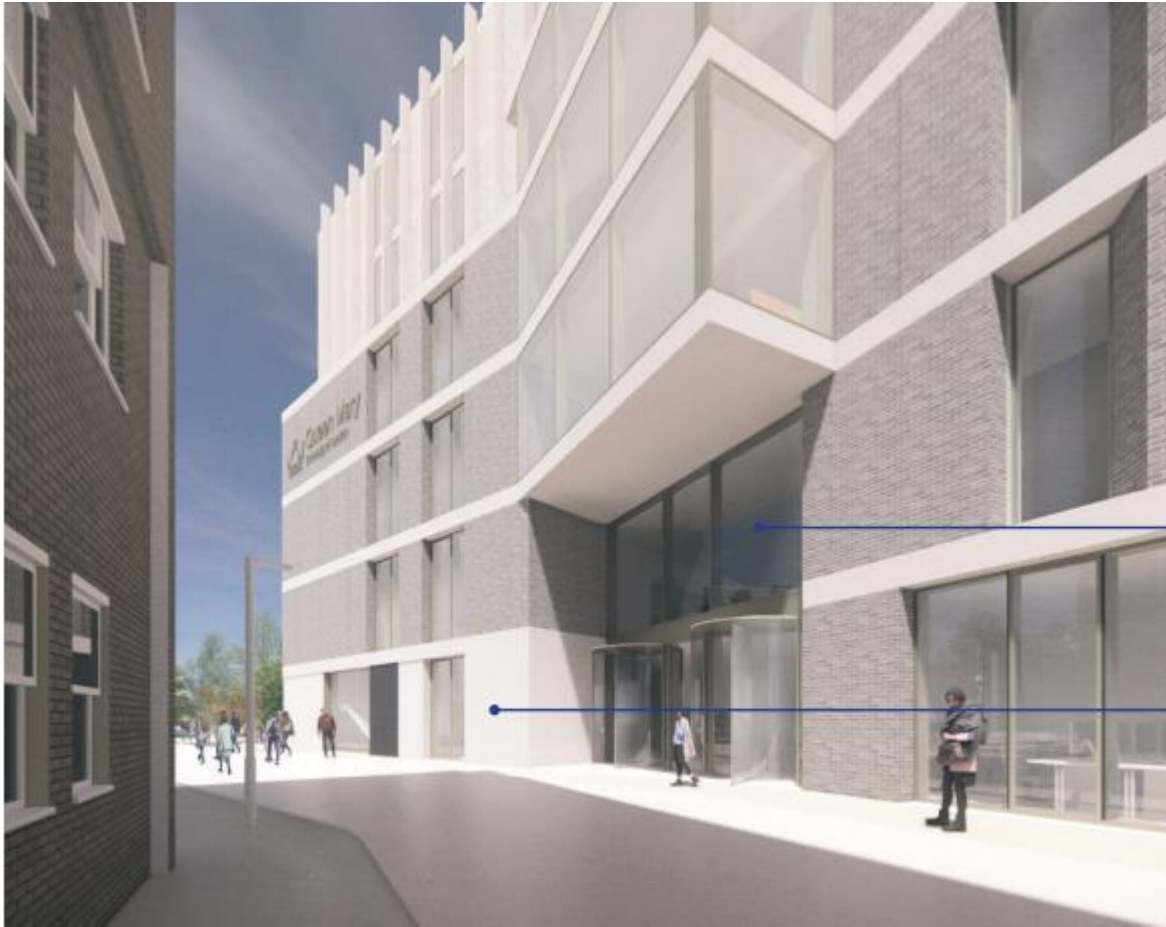
Building entrance from Westfield Way
