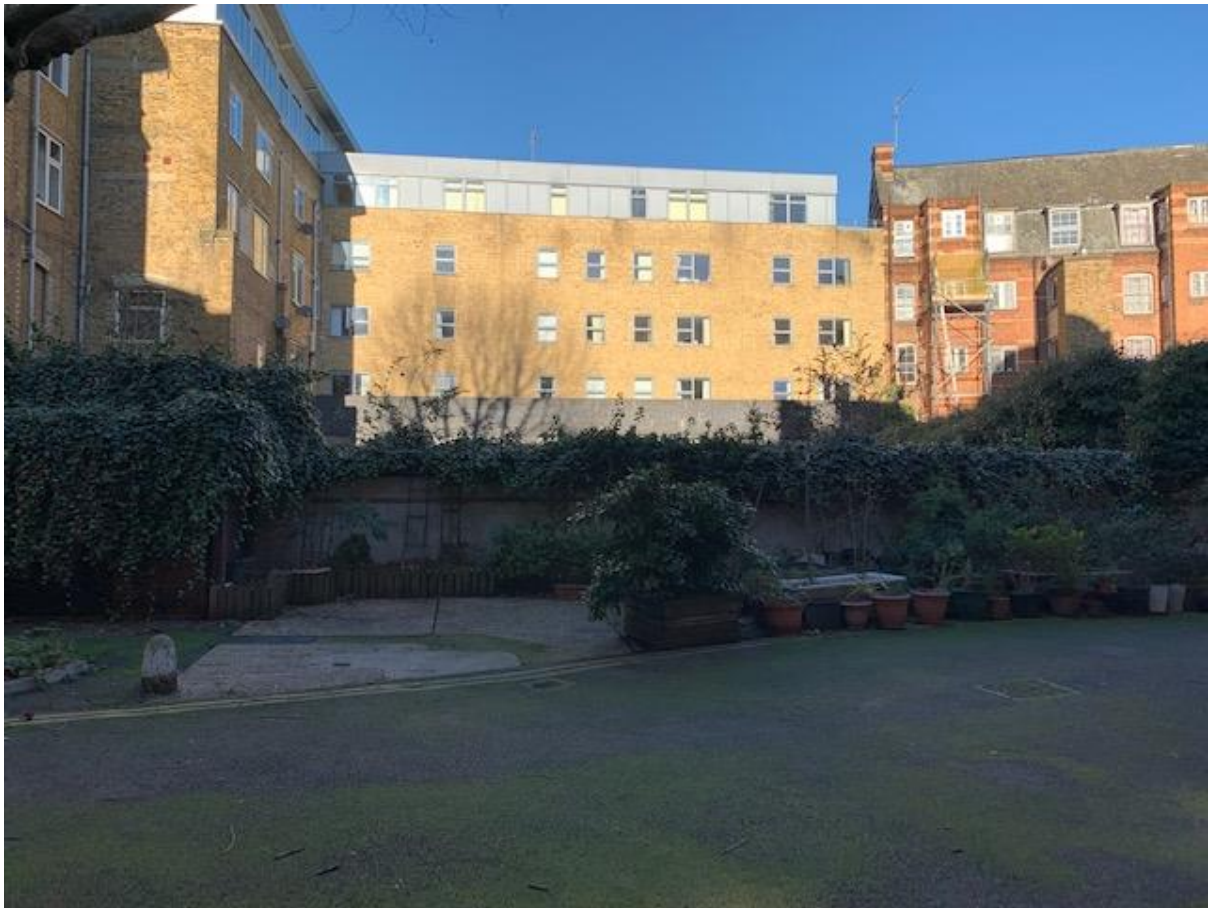
View of perimeter wall as existing from within Wargrave House amenity space with Leyton house in background
