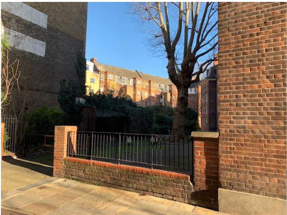
View from Boundary Street of perimeter wall with Walker House on left and Shipgrave House beyond
