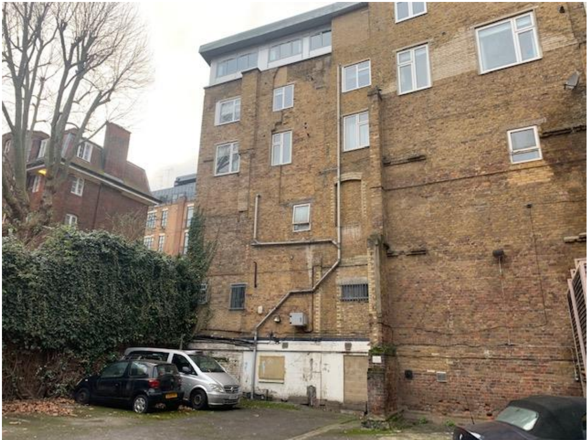
Rear of Walker House from Car Park
