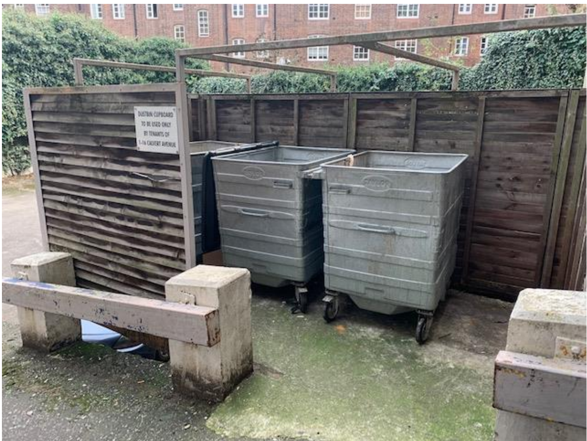
Existing refuse store serving 22 Calvert Avenue
