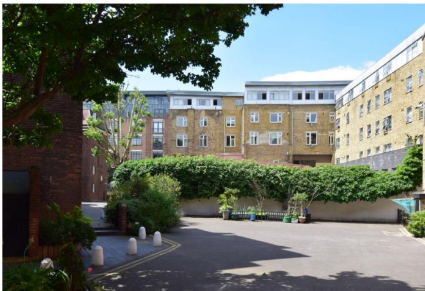
Figure 12: View of refused scheme from Shiplake House Courtyard
