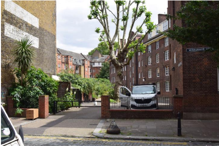
Figure 8: Existing view from Boundary Street.
