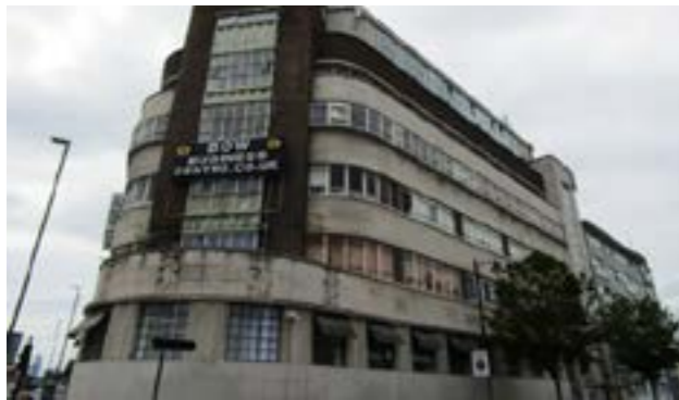
Fig. 15: Bow House Business Centre
