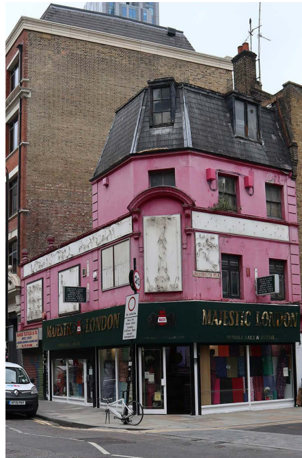
Redundant neon signage in high level bands and lower boards, No.1 Wentworth Street
