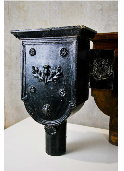
Decorative cast iron rainwater head / hopper
