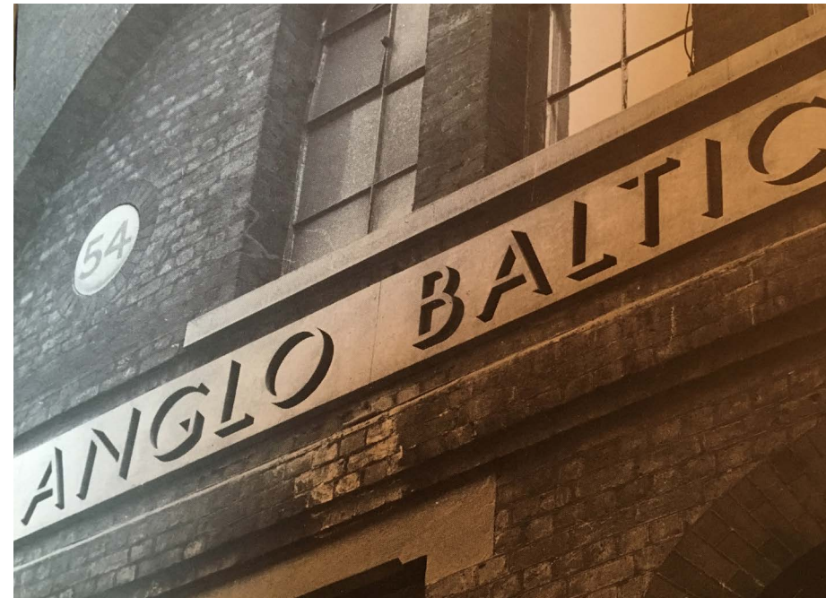
Contrasting band of signage on masonry building Location: unknown
