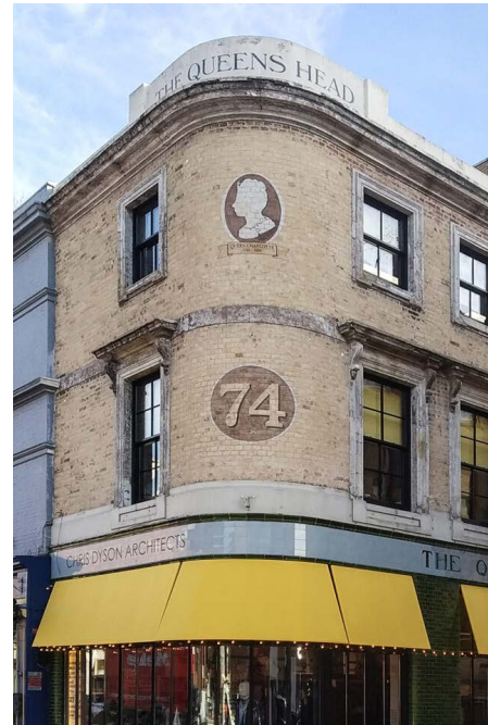
Hand painted signage on masonry Chris Dyson Architects, Commercial St
