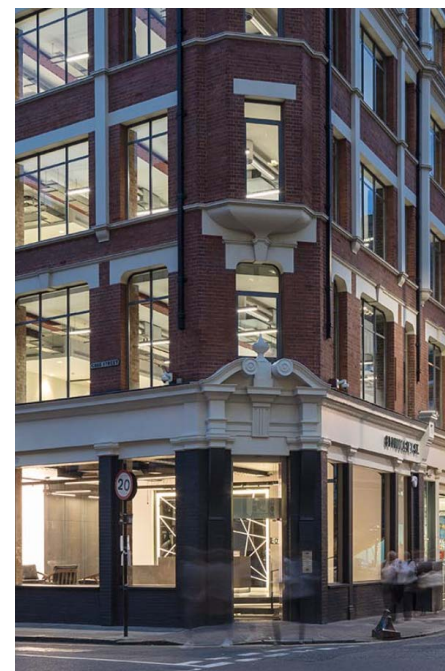
80 Middlesex Street Downpipe running inside building at first floor level
