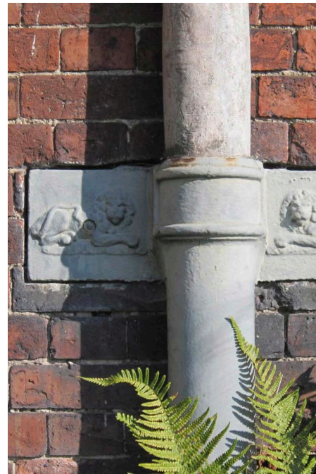
Decorative brackets rebated into brickwork
