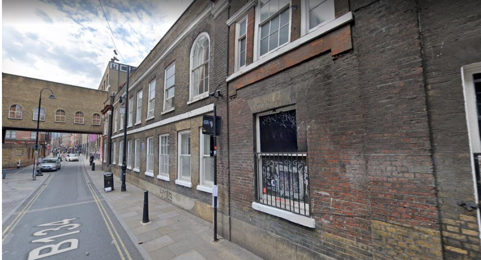
Figure 23: Street view image of grade II * listed Directors House (right), looking south along Brick Lane
