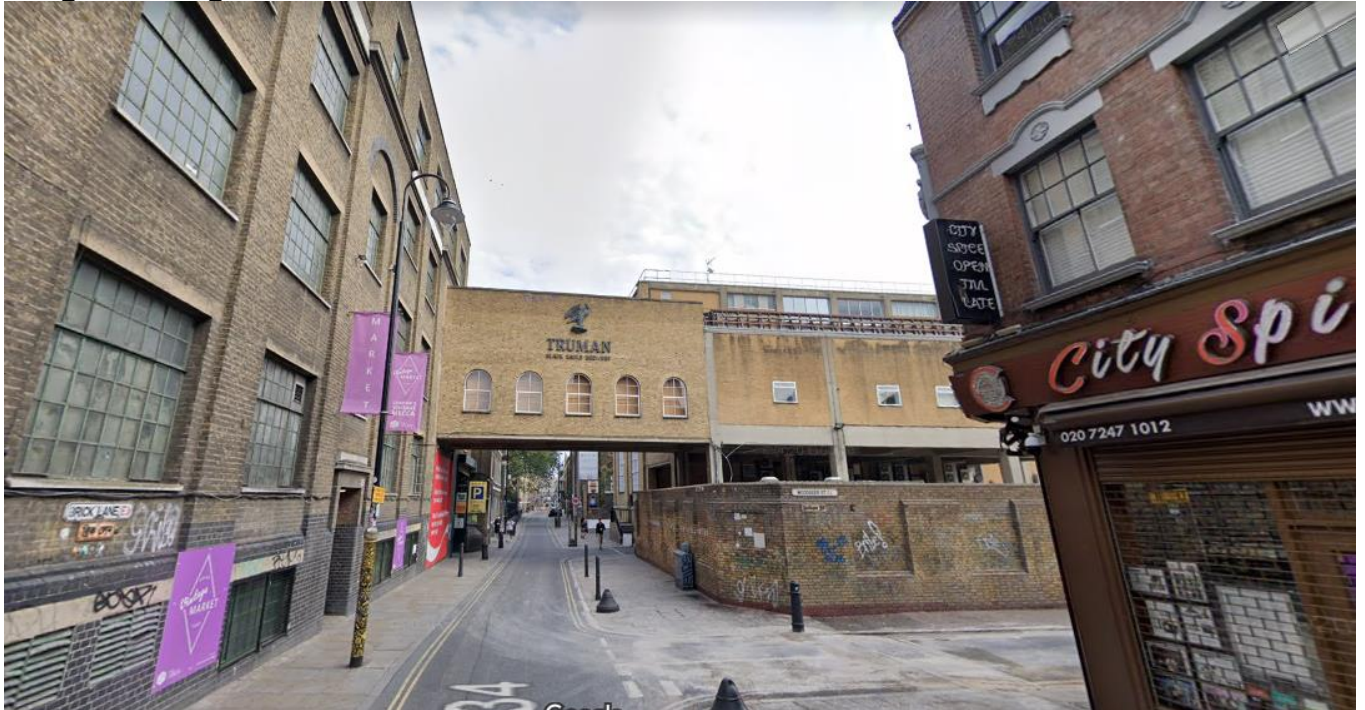
Figure A: View looking north along Brick Lane; the wall bounding Plot S1 (on the application site) is shown on the right; Block F is shown on the left; the Truman's bridge crossing Brick Lane in the centre of the view.
