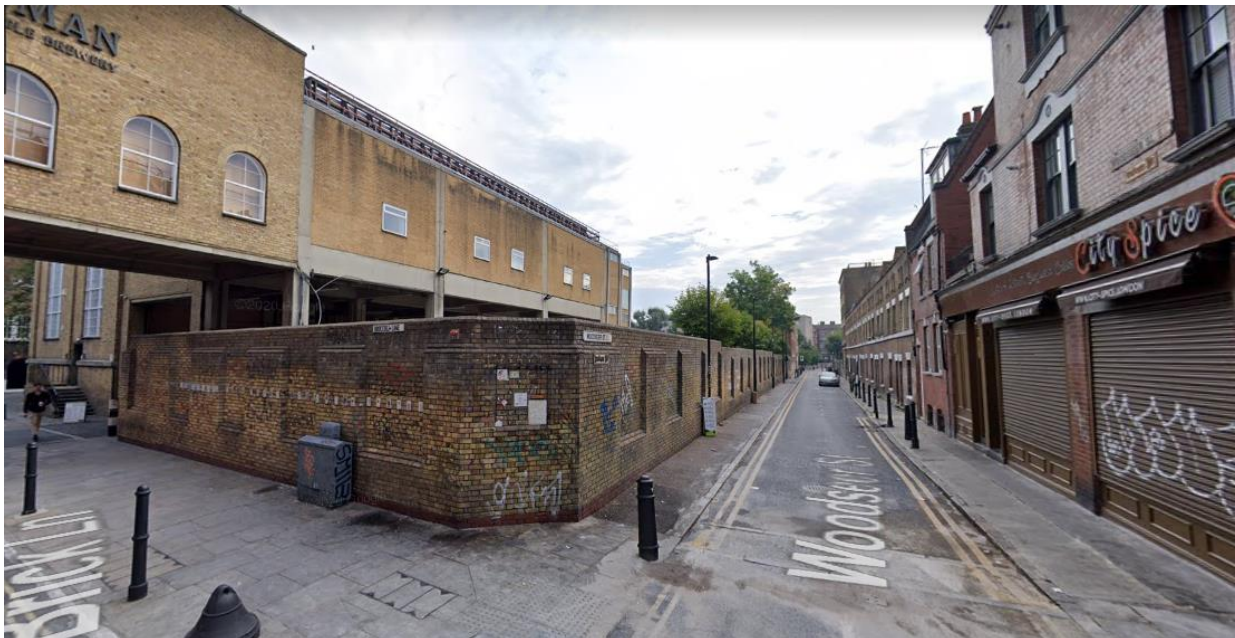
Figure 5: Street view of the corner of Brick Lane and Woodseer Street (existing)
