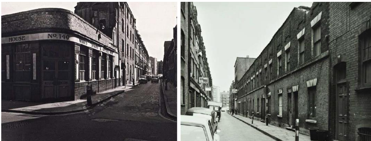
Figure 25: Left: Views looking east down Woodseer Street circa 1975 showing the Black Eagle Tap public house on the corner of Brick Lane and terrace development on the north side of the street
