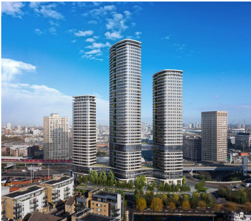
Figure 7 - View looking north
