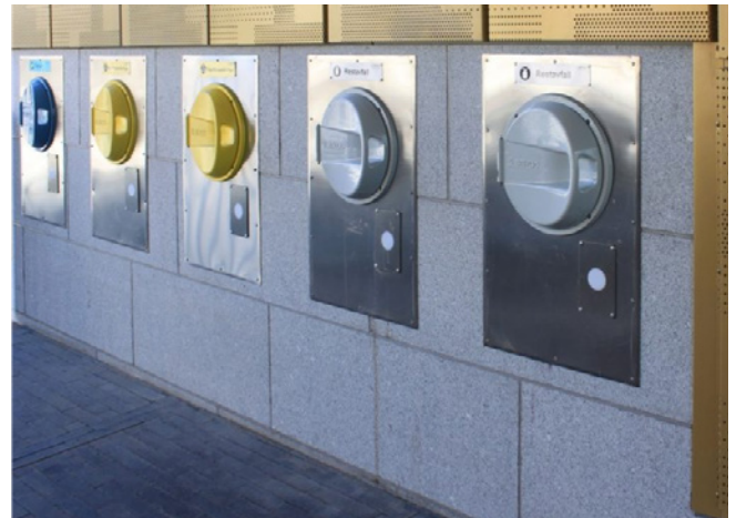
Fig. 14. An example of an AWCS portal area, demonstrating ease of access. Image courtesy of Envac.
