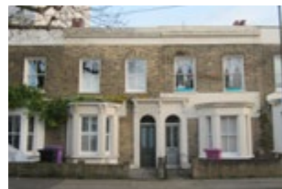
B. Late 1860s 2-storey terraces with canted bay window at ground floor and simple Victorian sash windows above, stuccoed details on ground floor, part of Swaton Road Conservation area.
