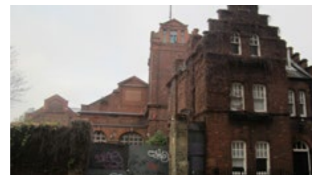
The Grade II* listed former Wapping Hydraulic Pumping Station from 1893, within the Wapping Wall Conservation Area.
