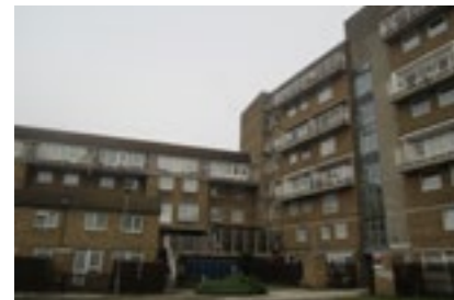
A. The post-war Glamis Estate (East), one of the last major estates built by the Greater London Council in the 1970s. It displays a concern for a more human scale with blocks of pale brick with up to 8 storeys. One terrace includes projecting glazed stair walls.
