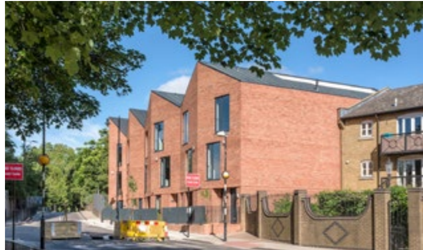
Old Ford Road London (Tower Hamlets) pH+ Architects
