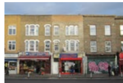
G. Terrace with ground floor shops and varying window treatments on Burdett Road, within the Ropery Street Conservation Area.
