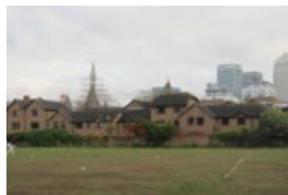
B. Self-built row of houses built between 1987-1989 in pale brown-black brick and pitched/hipped roofs influenced by the materials of St. Saviours Church and its former vicarage, which the houses surround.
