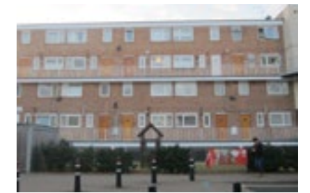
F. The post-war Bede Estate. The majority of the estate was built between 1964-1971 and comprises primarily 4-storey brick units made up of deck-access maisonettes.
