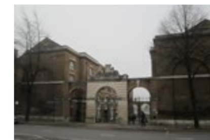
H. Free Trade Wharf built in 1796 on the Thames Path, within the Wapping Wall Conservation Area. The warehouses were converted into offices and residences in 1987. It is of yellow brick, 9 bays with a 10th bay expressed as a pedimented 2-storey pavilion.
