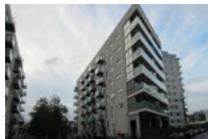
A. Mixed-height linear blocks of up to 10 storeys built in the 2010s, with views facing towards Limehouse Cut.
