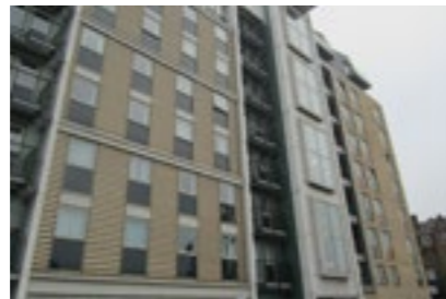
B. Student housing development for Goldsmiths University students on King David Lane built in 2009-2010, with up to 8 storeys and balconies for each floor.
