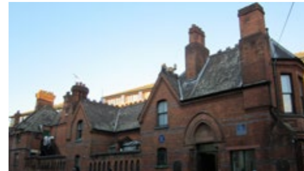
The Grade II listed former Bryant and May Factory, now a residential development.
