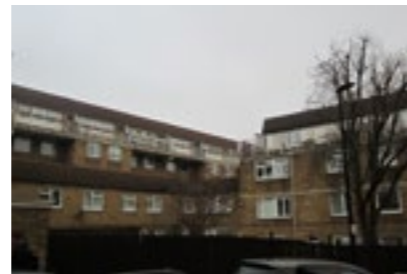
C. The post-war Glamis Estate (West), one of the last major estates built by the Greater London Council in the 1970s. It comprises 2-3 storey blocks with deck-access and courtyards, and a 22-storey tower block.
