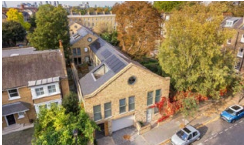
Tredegar Square London (Tower Hamlets) Jonathan Freegard Architects
