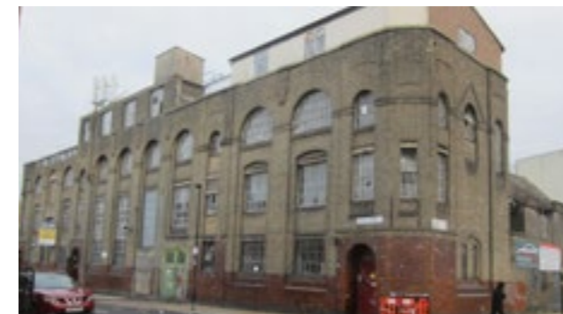
Former stock brick Factory from 1911, within the Brickfield Gardens Conservation Area.
