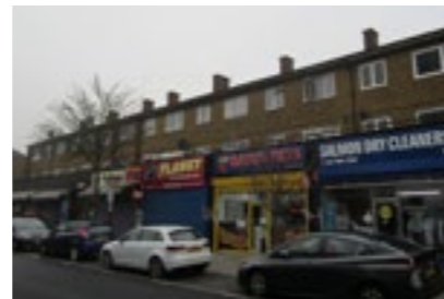
C. Post-war 3-storey blocks of flats with balconies extending over shops, built in 1958 on Salmon Lane as part of the Locksley Estate.
