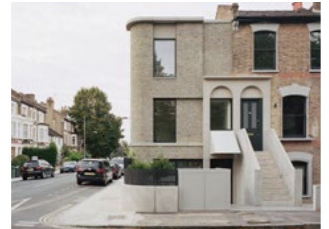
Building on the corner that incorporates the same proportions for windows, doors and stairway access of terrace in its contemporary design approach. (photo ©Rory Gardiner)
