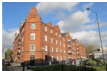
B. Cressy House, a mansion block built in 1894 as a 4-storey housing development commissioned by East End Dwellings Company.
