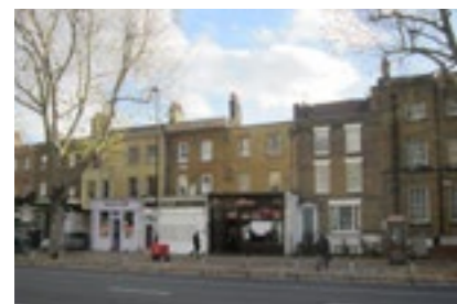
A. Long terraces along Mile End Road with a continuous building line and varying heights, most of them with commercial ground floor and 2-storeys residential above dating from early 19th Century.
