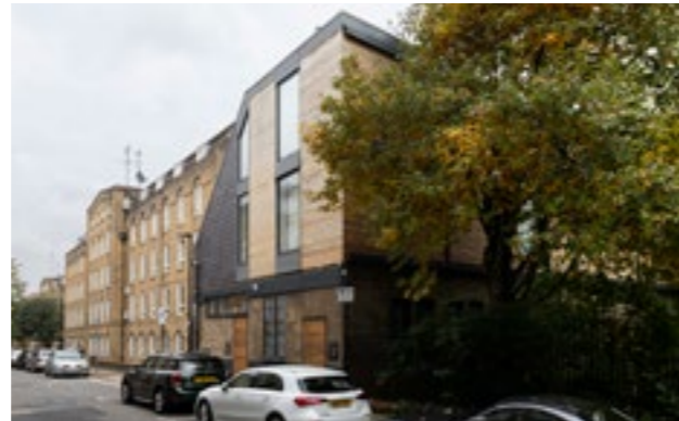
Slate wall tiles and timber cladding respond well to surrounding industrial character and brick façades. Good detailing have ensured that the cladding materials have weathered well. (photo ©Ivan Jones)
