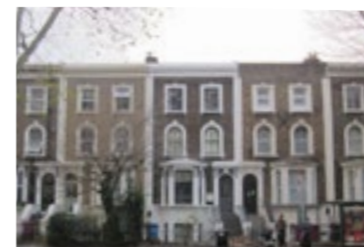
G. Late 19th Century grand terraces with elevated ground floor, semi-basements, 3-sided bay windows and decorative stuccoes surrounds to windows and doors, remnants of the Cotton Estate, now part of the Brickfield Conservation Area
