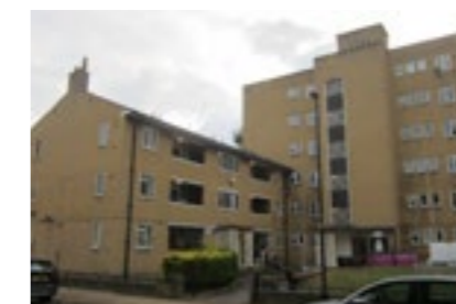
H. Mix of 3- and 6-storey blocks completed in 1951 and built with London stock brick and slate to reflect the existing housing stock of the area at the time, part of Lansbury Conservation Area.
