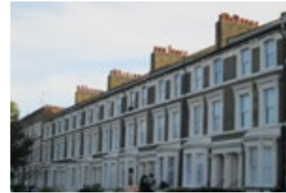
D. Terraces of Italianate houses from circa 1865, on Old Ford Road, within the Victoria Park Conservation Area. They have paired doorways in flat arches on composite, engaged columns.
