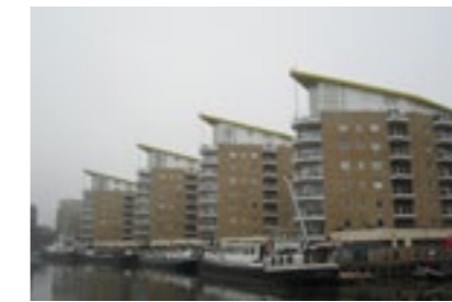
E. Residential towers completed in 1998 as part of Basin Approach, a residential development around Limehouse Basin. The four blocks are of 8 storeys with the upper one of double-height. It is of brick with projecting balconies onto the basin.
