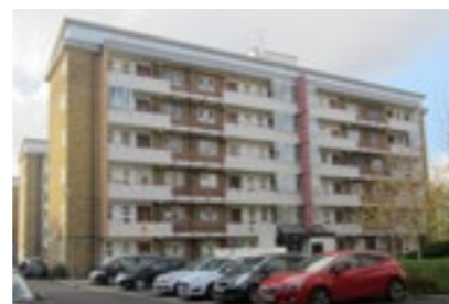
C. Post-war 1960s housing estate part of Ocean estate North, one of 6-storey blocks with continuous deck-access.
