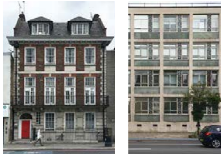
Existing facades fronting Mile End Road, Albert Stern House (left) and the Engineering Building (right)
