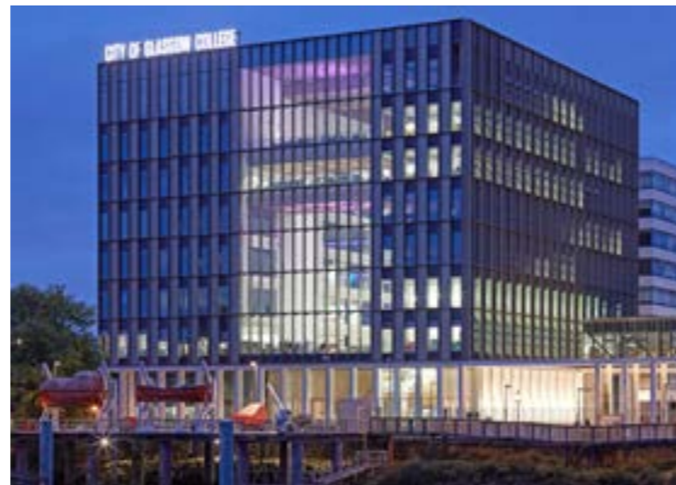
Precedent image: Circulation atrium brings interest to the facade while allowing light into deep plan
