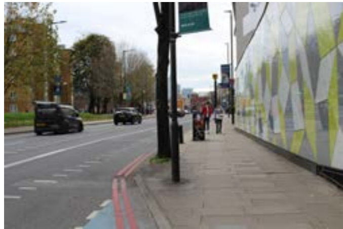
Existing blank facades on Mile End Road
