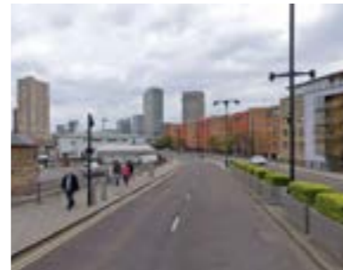
View north along Trafalgar way with the Billingsgate market site on the left and existing medium-density residential context on the right
