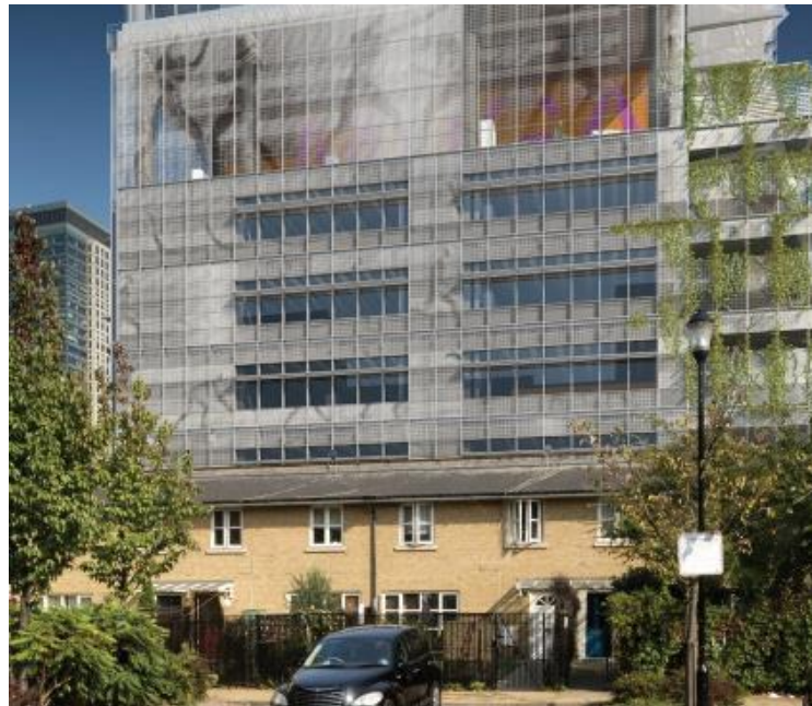
Bellamy Close looking east with Alpha Square development in the background.
