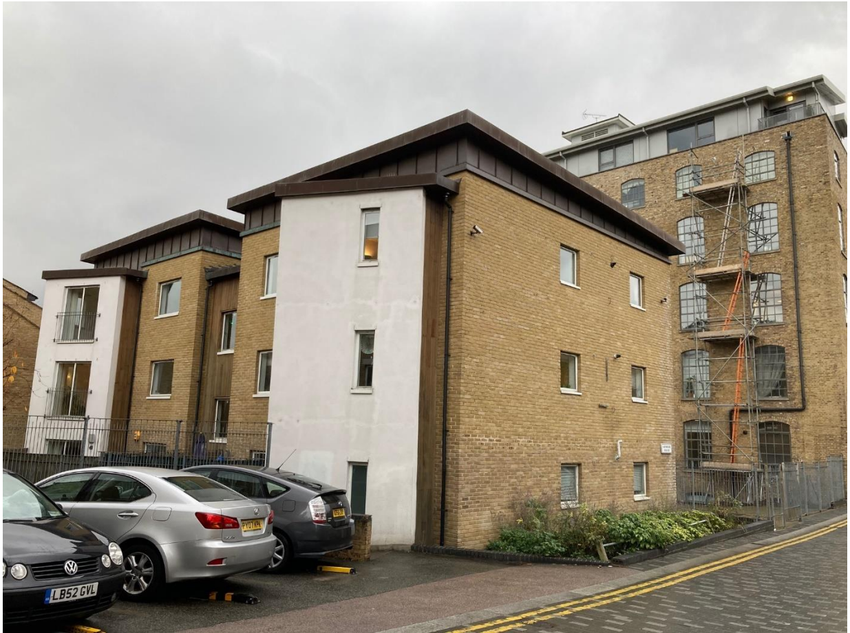
Figure 5: The site from Gunmakers Lane looking south east with Albany Works to the south
