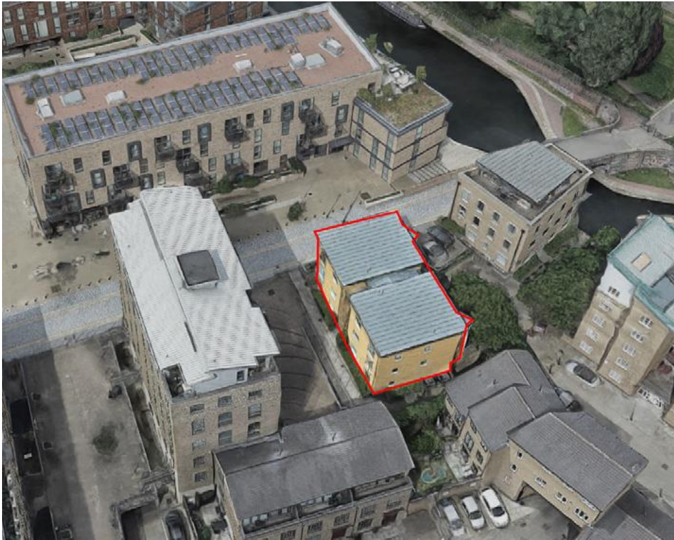
Figure 1: Site and surrounding buildings
