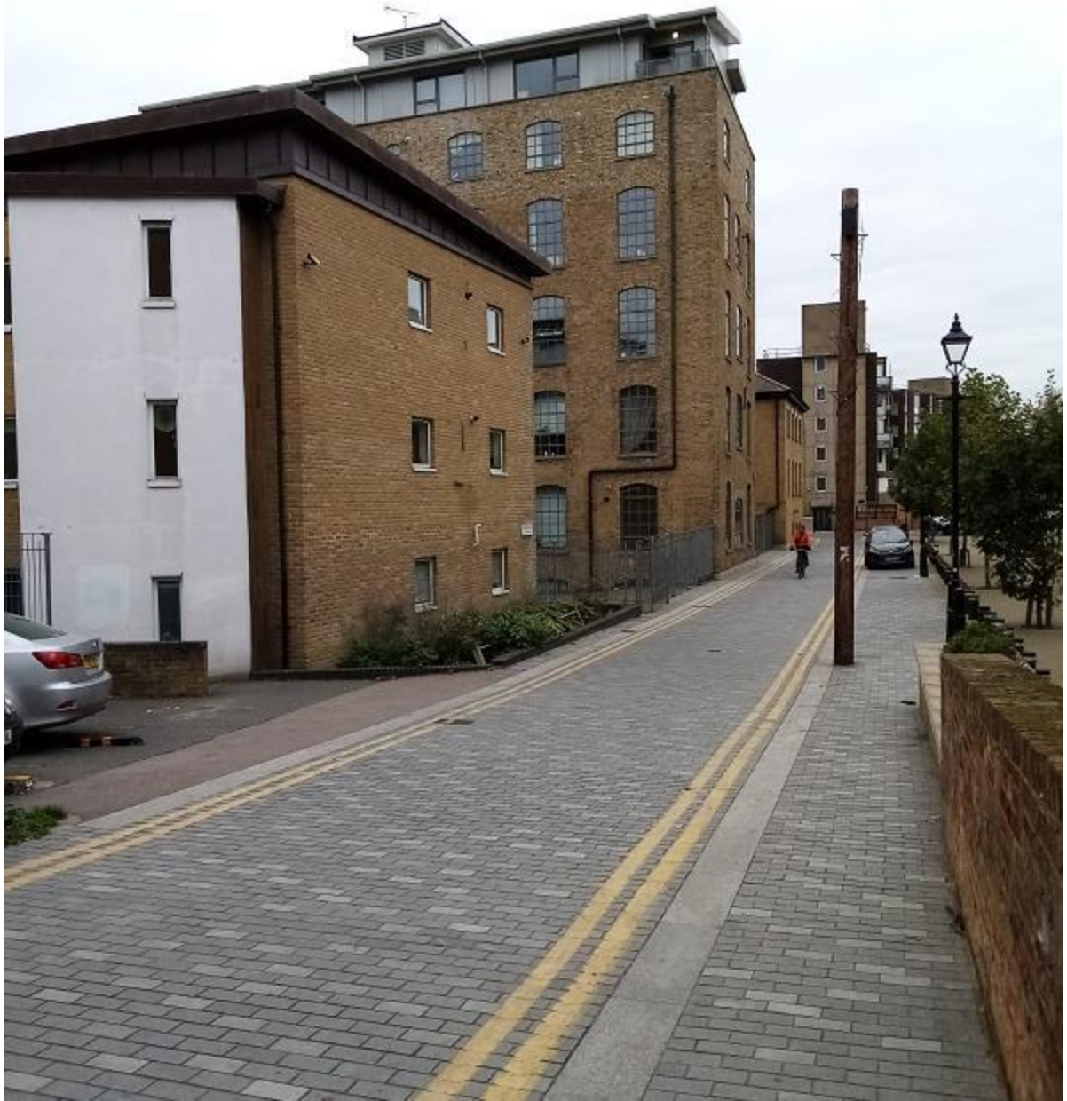
Figure 6: A view looking down Gunmakers lane from the south end of Three Colt Bridge
