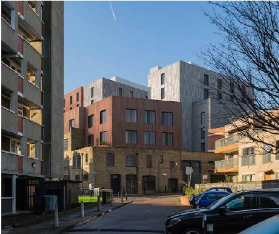
Figure 9 Diss Street building elevation viewed from south of Stamp Place
