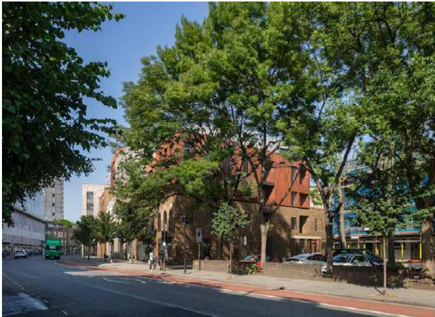
Figure 8 South facing flank wall, Hackney Road junction with Pelter Street (residential block)
