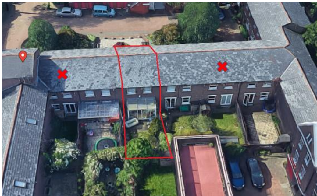
Figure 4: Rear elevation of the terrace
