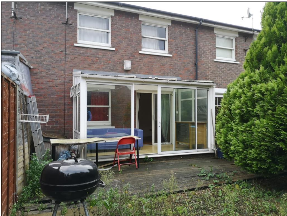
Figure 2: Rear elevation of the application site
