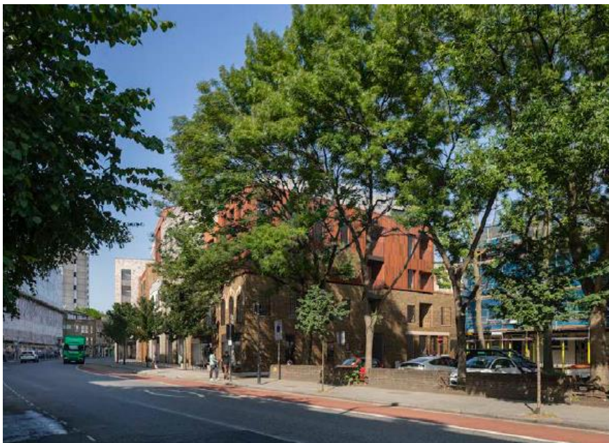
Figure 8 South facing flank wall, Hackney Road junction with Pelter Street (residential block)
