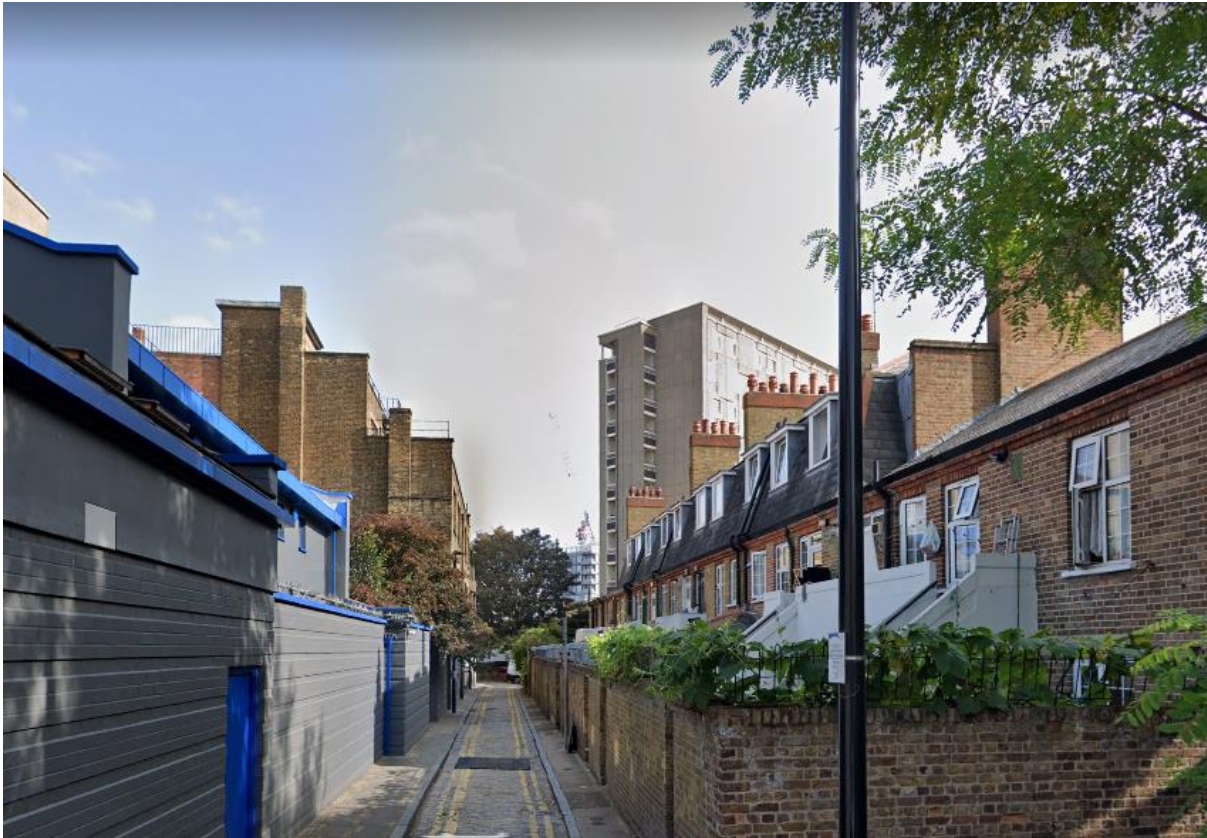
Figure 5 Pelter Street: Existing building rear elevation far left and properties at 1-14 Vaughan Estate to the right. In grey and blue, the existing medical centre on Strouts Place junction with Pelter Street
