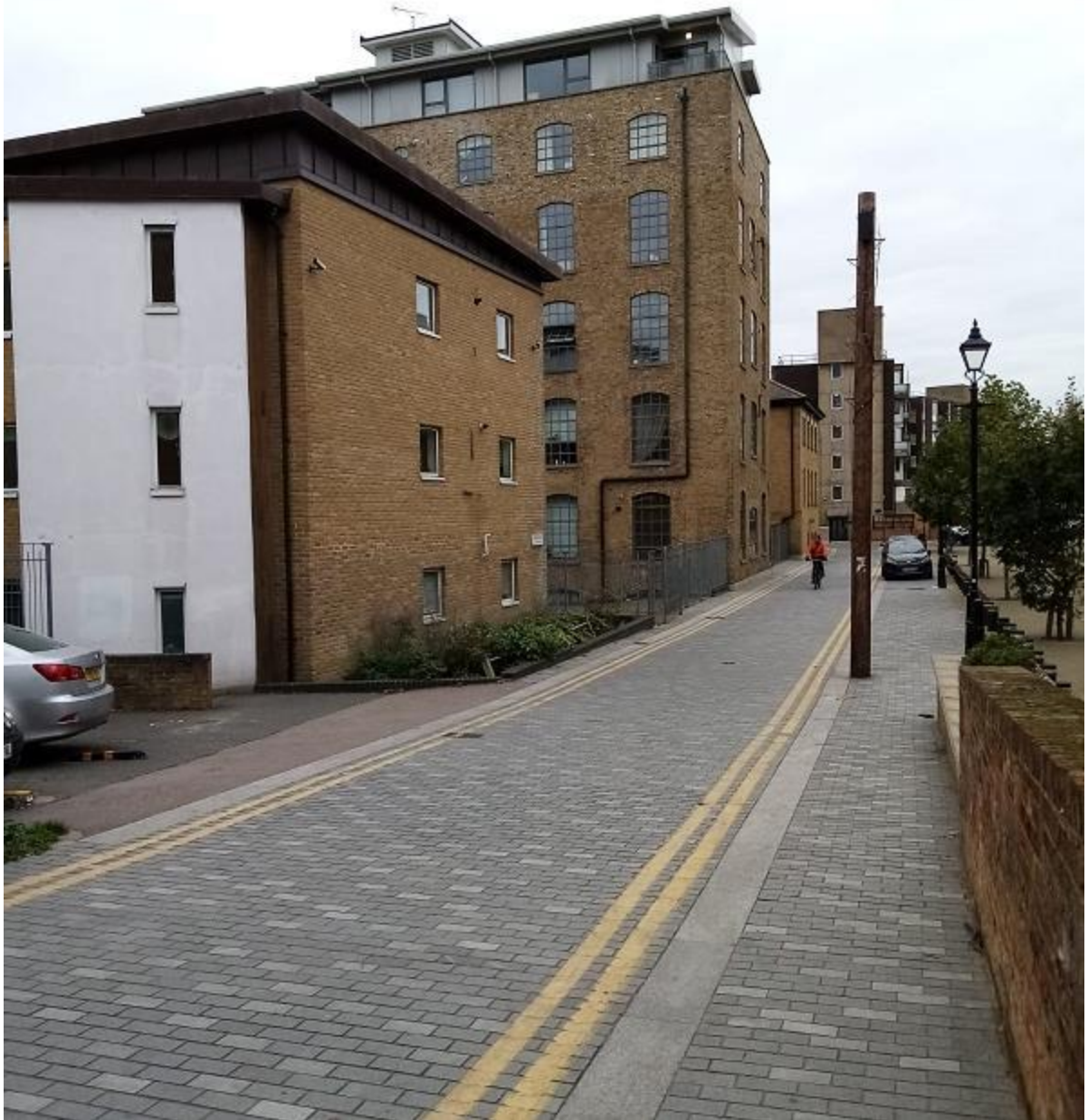
Figure 6: A view looking down Gunmakers lane from the south end of Three Colt Bridge
