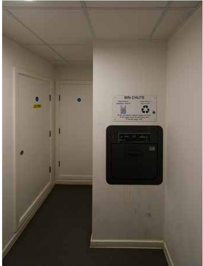
An ineffective waste chute. It is not located in a special room, signage is unclear, the area lacks ventilation and the surrounding area would be easily damaged if waste was left on the floor.
