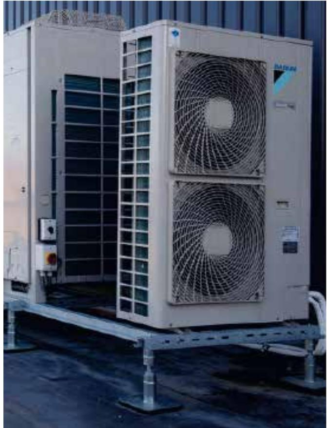
Air source heat pumps can be located on the topmost rooftops.
