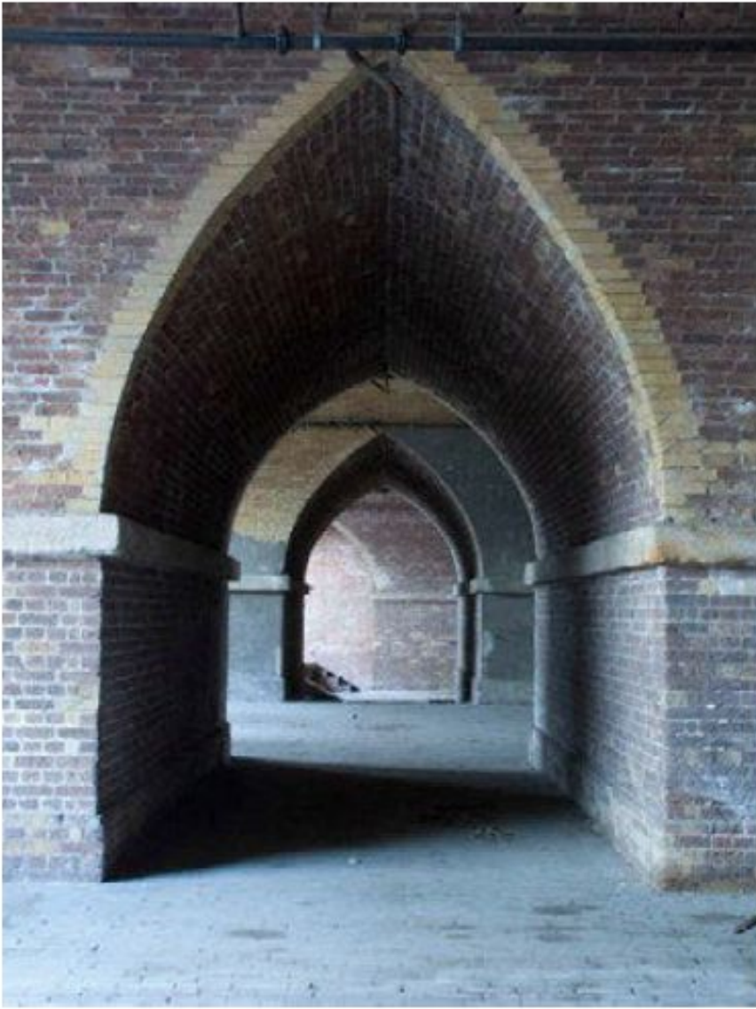
Figure 13: Existing photograph of listed arches under Braithwaite Viaduct
