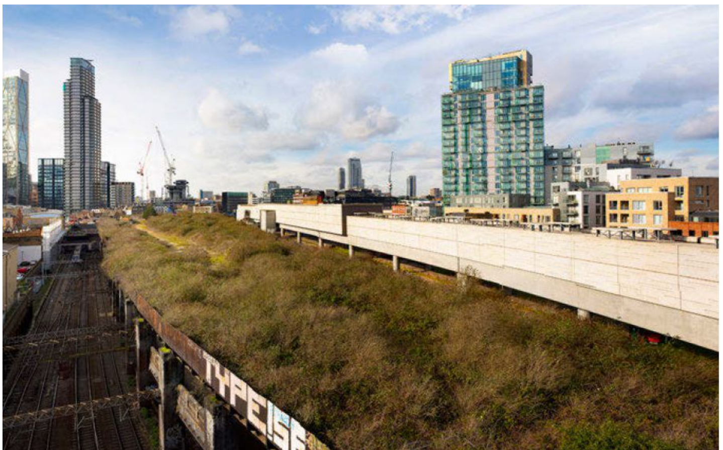
Figure 8: Existing photograph of platform level above Braithwaite Viaduct from the east end of site looking west.
