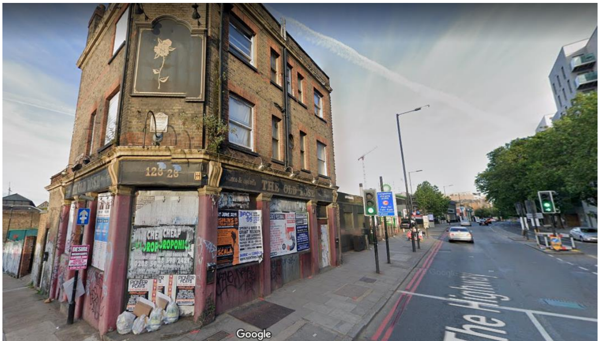
Figure 3: View of application site from the north-east on The Highway (The Old Rose on the left) (Google)
