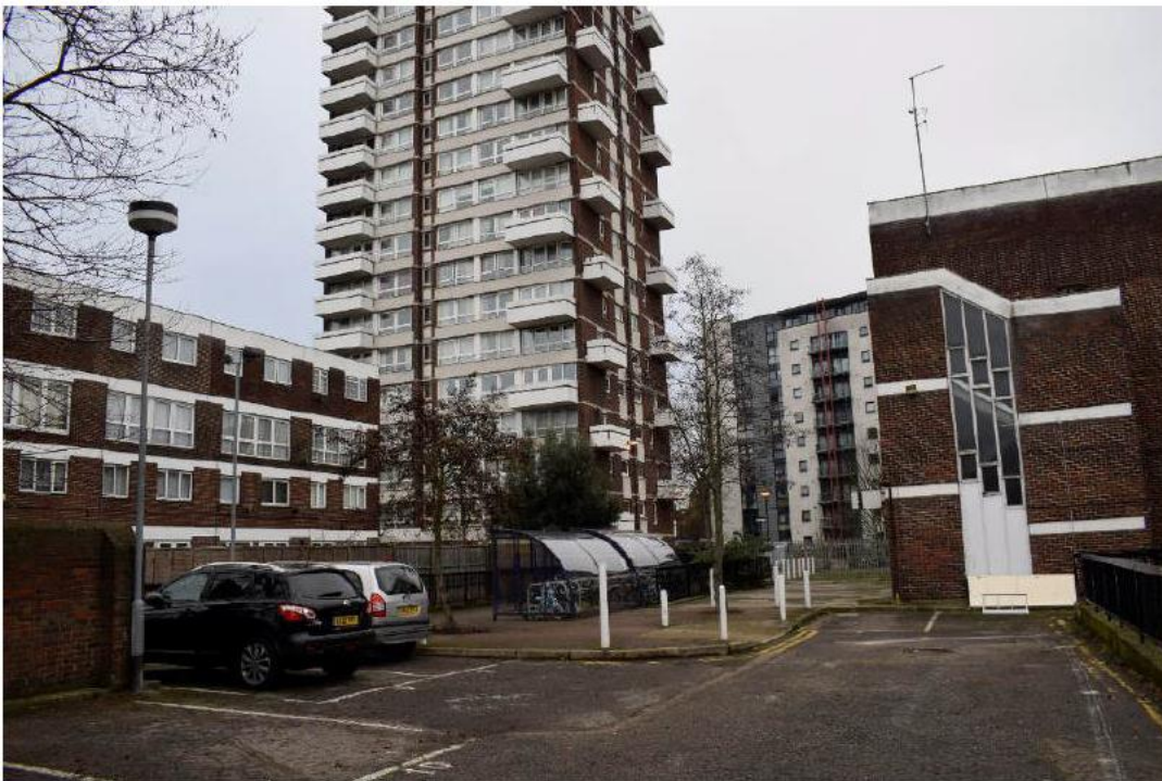
Figure 4 : Existing Buildings within the Estate
