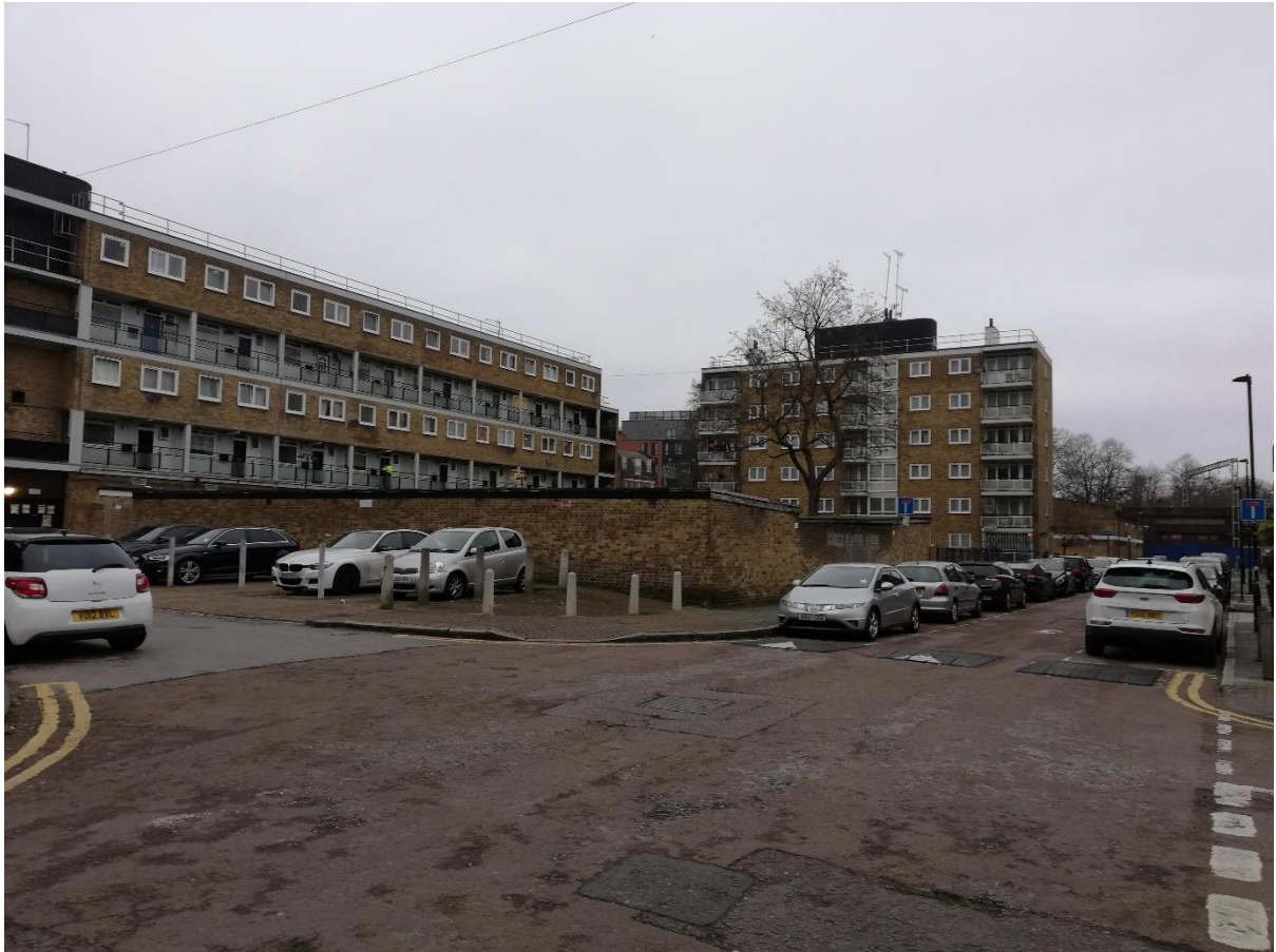
Existing site – photo of existing single story garages looking north west from Wickford Street (64-134 Cambridge Road and Frederick Charrington House in the background)
