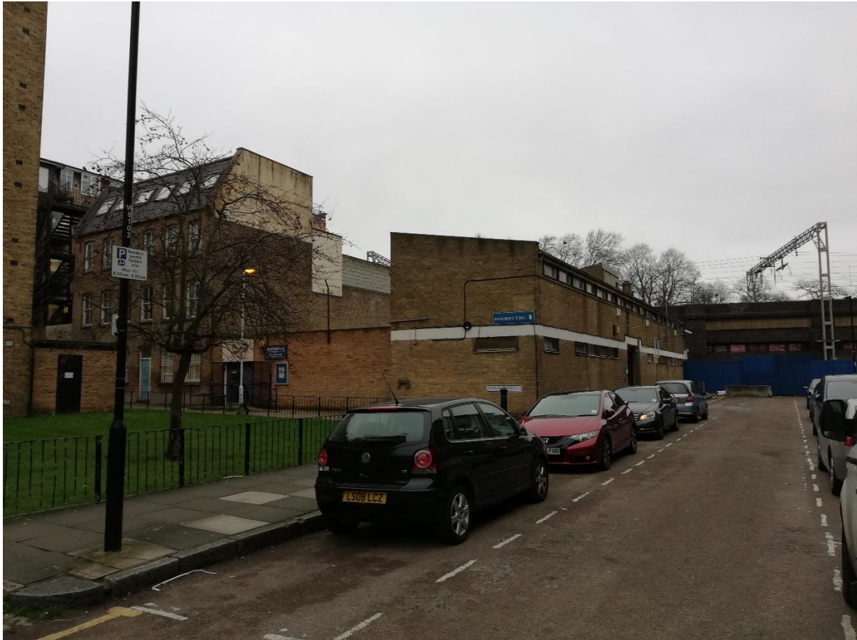
Existing site – photo of existing Bancroft TMC building looking north from Wickford Street Lane
