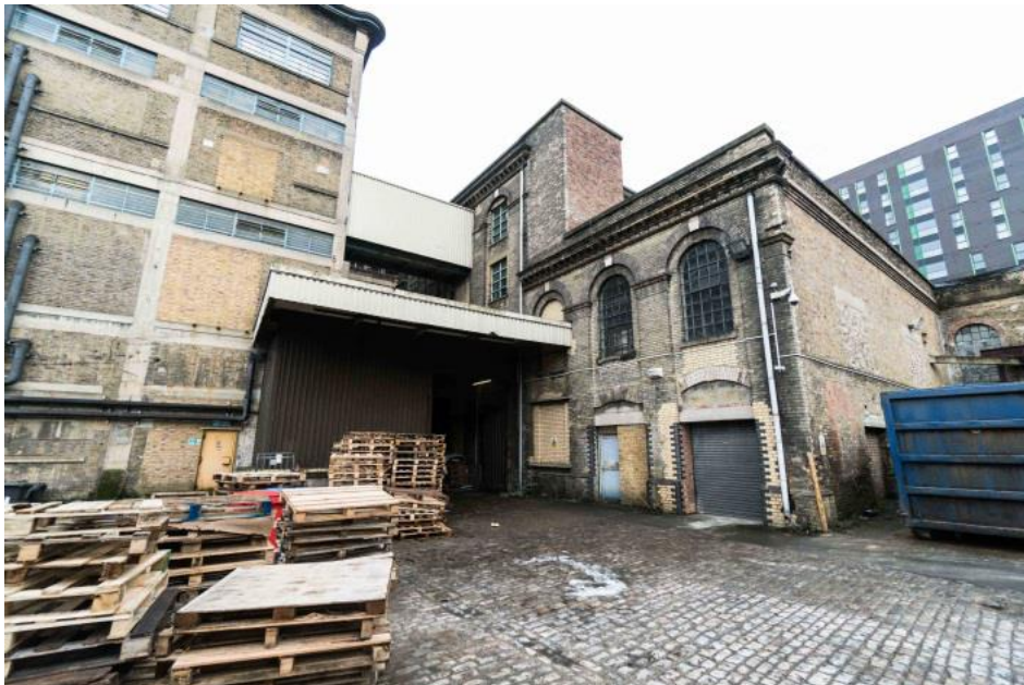
Northern service yard
