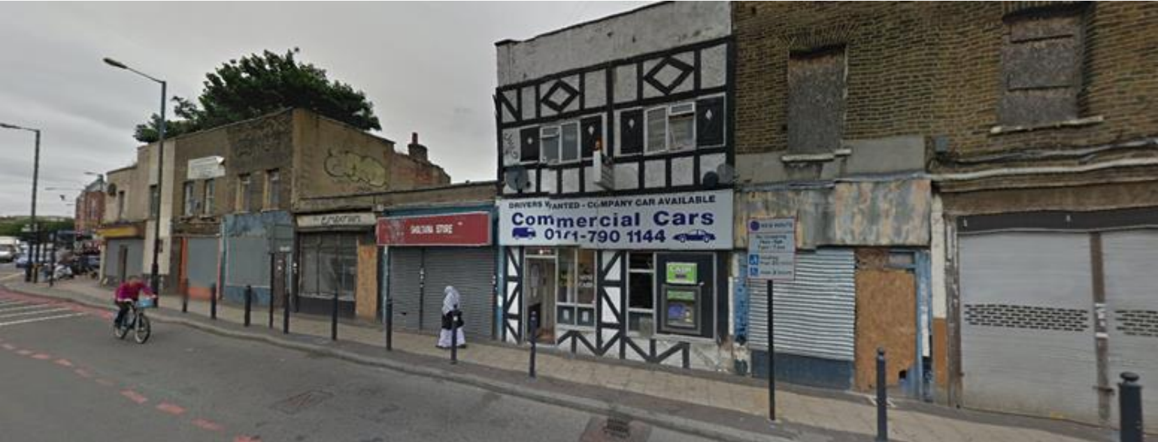
Existing site – View of no. 605 – 621 Commercial Road looking north west (prior to demolition)
