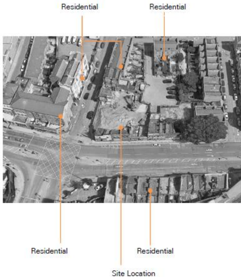
Figure 6 – Subject Site and Surrounding Developments
