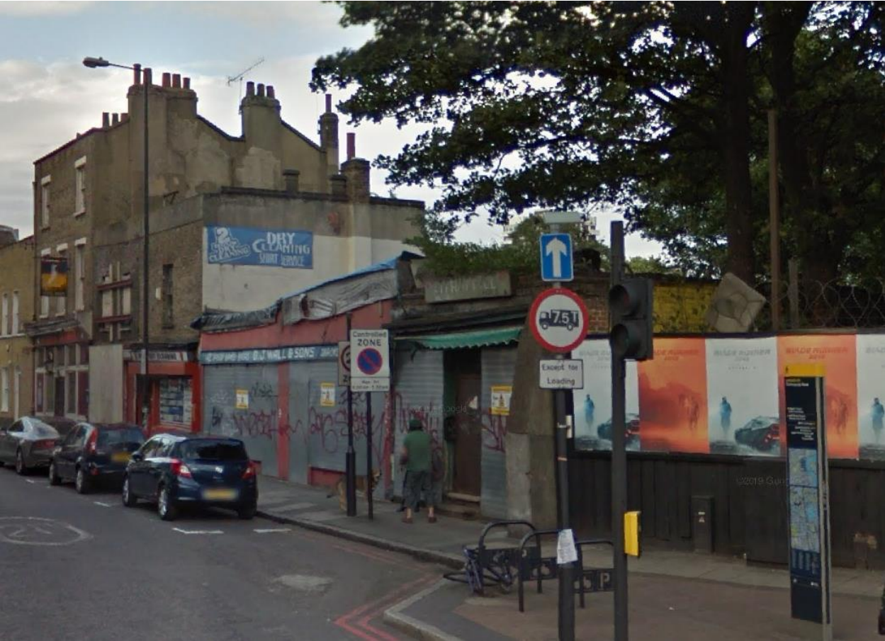
Existing site – View of nos. 44, 46 and 48 White Horse Road (prior to demolition)
