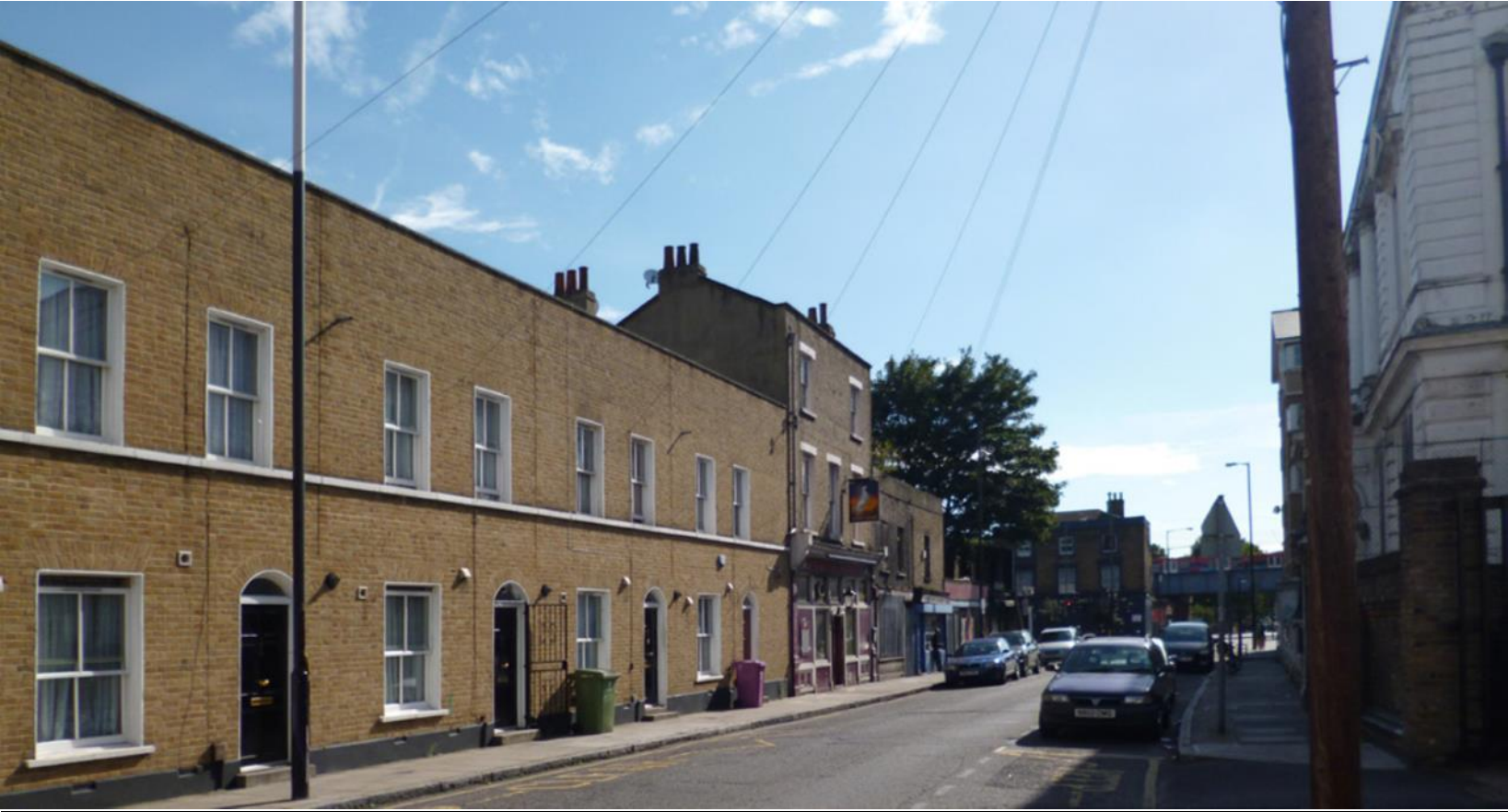
Existing site – View from White Horse Road looking south (prior to demolition)
