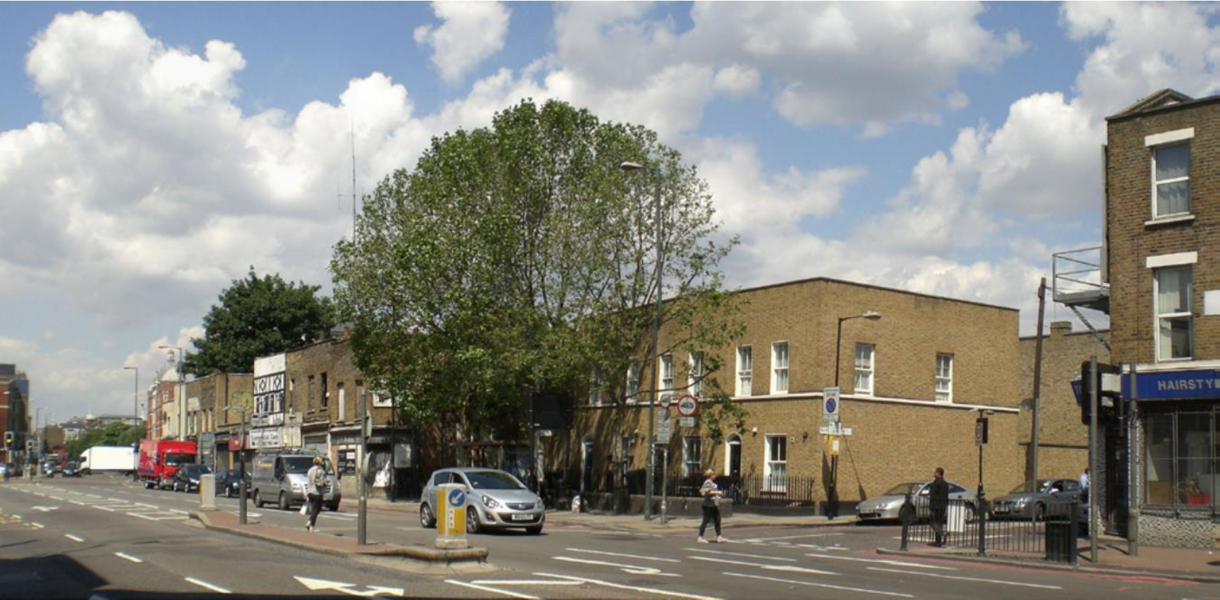
Existing site – View from Commercial Road looking north west (prior to demolition)
