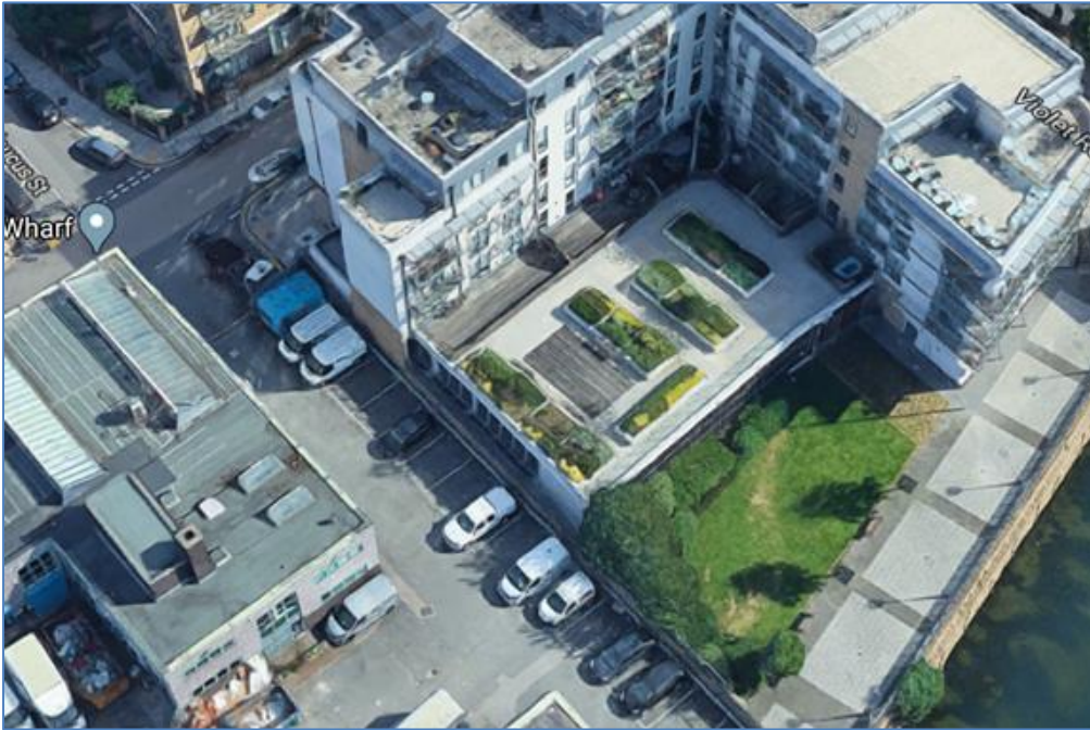
Figure 5 - Aerial photograph showing the Caspian Wharf podium terrace
