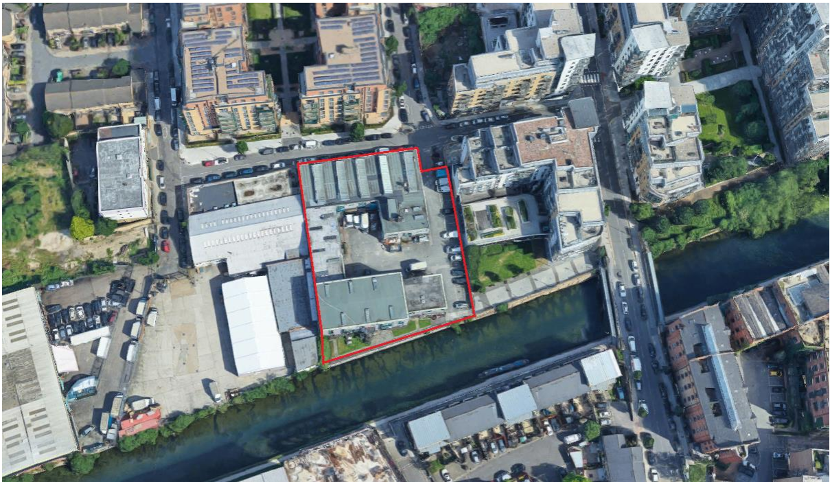
Aerial view of the site and surroundings
