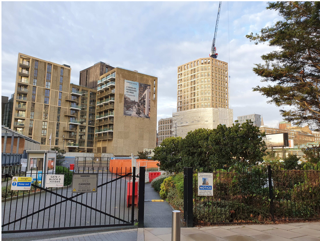
View from Virginia Street into the site (west direction from Virginia Street)
