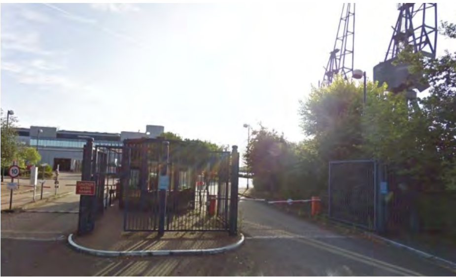
Entrance to Westferry printworks site on Isle of Dogs after being flattened for redevelopment. Picture source: Google
