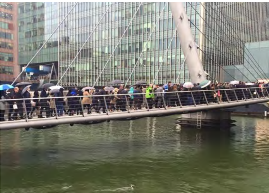
Congested old footbridge crammed with commuters queuing to reach Canary Wharf Underground station. Picture: Sergey Kharlamov
