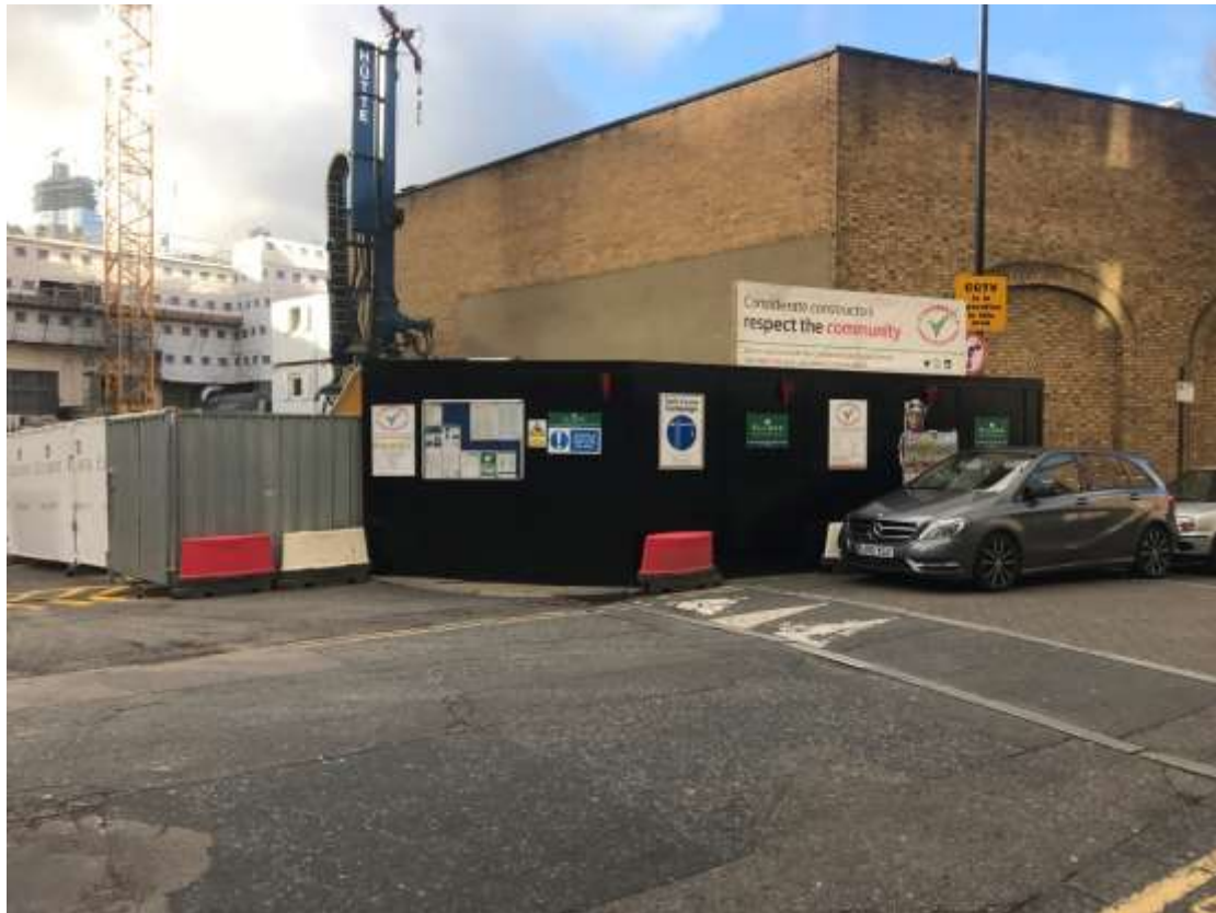
Existing elevation as seen from Fieldgate Street. The building to the right is the 1980s extension and to the vacant part of the sites are to the left
