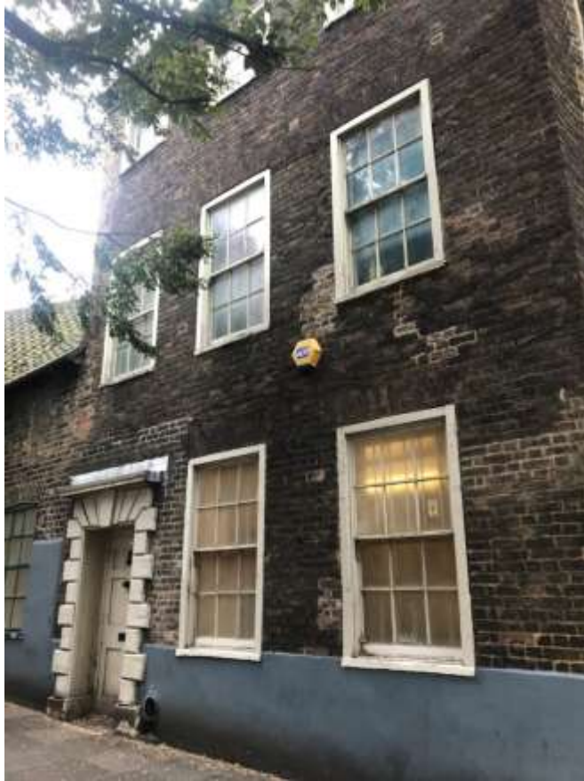
Close up of existing elevation along Whitechapel Road
