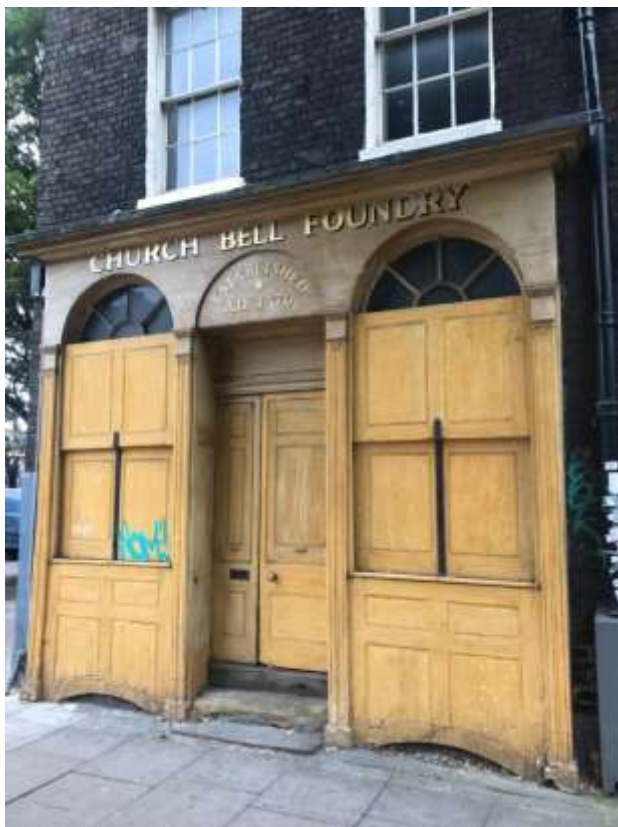
View of existing entrance from Whitechapel Road
