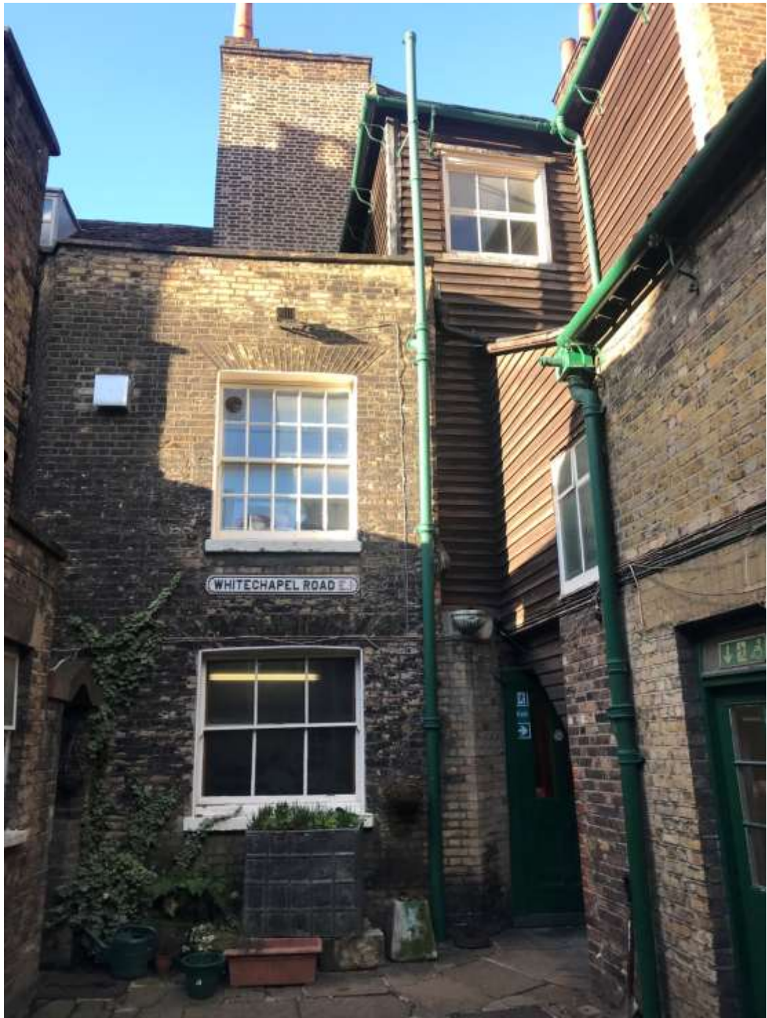
View of internal courtyard within existing foundry (facing north towards Whitechapel Road)
