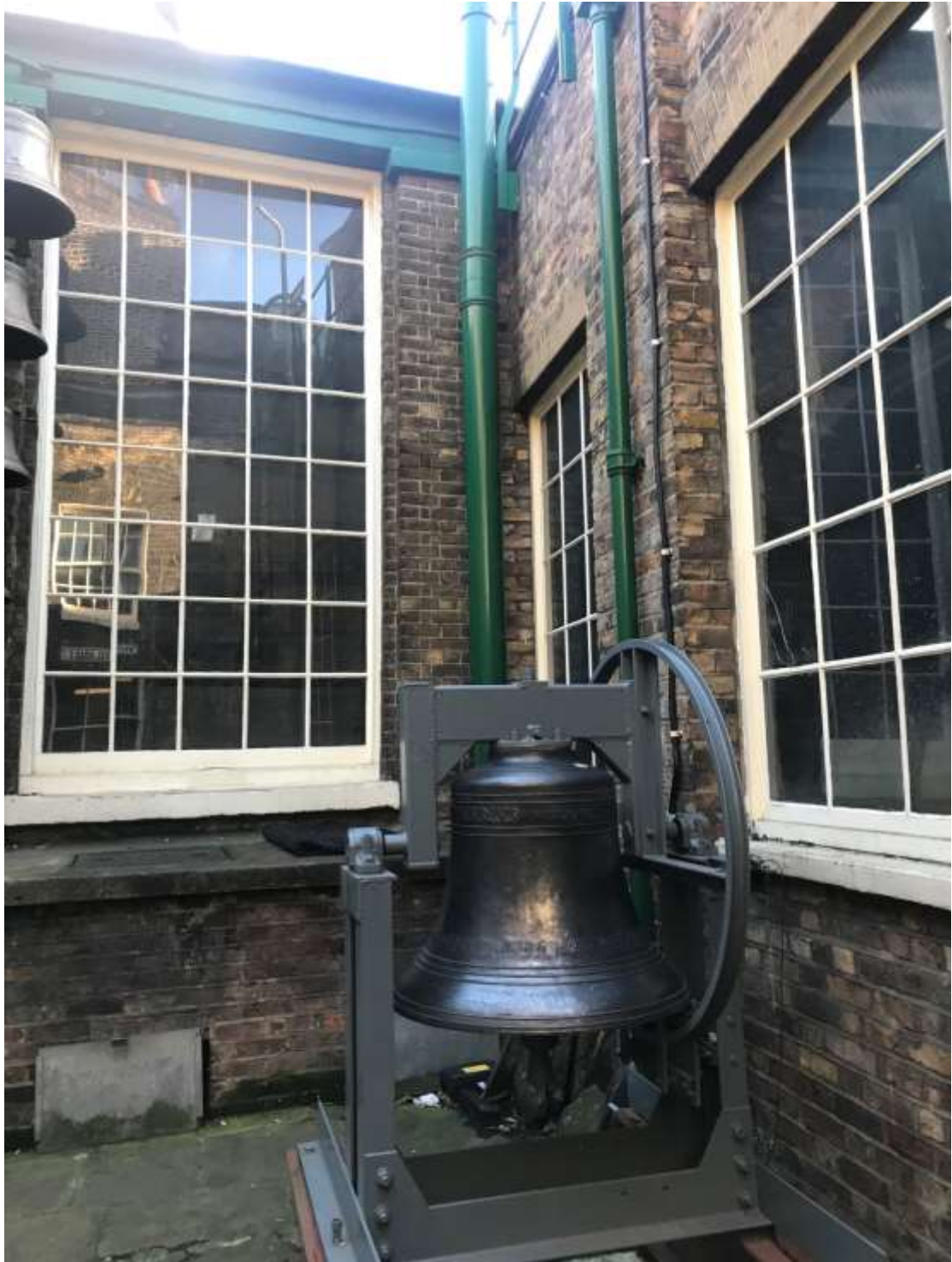
View on internal courtyard within foundry (facing south towards the 1980s extension and Mulberry Street)
