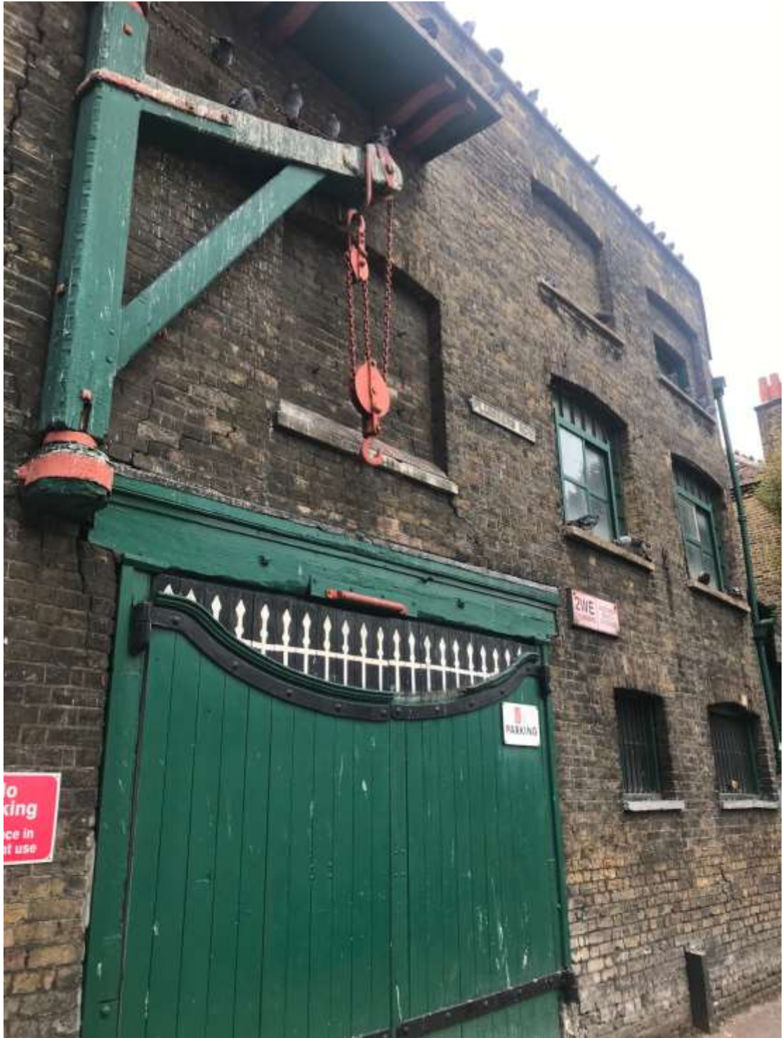
Existing close up of elevation on Fieldgate Street
