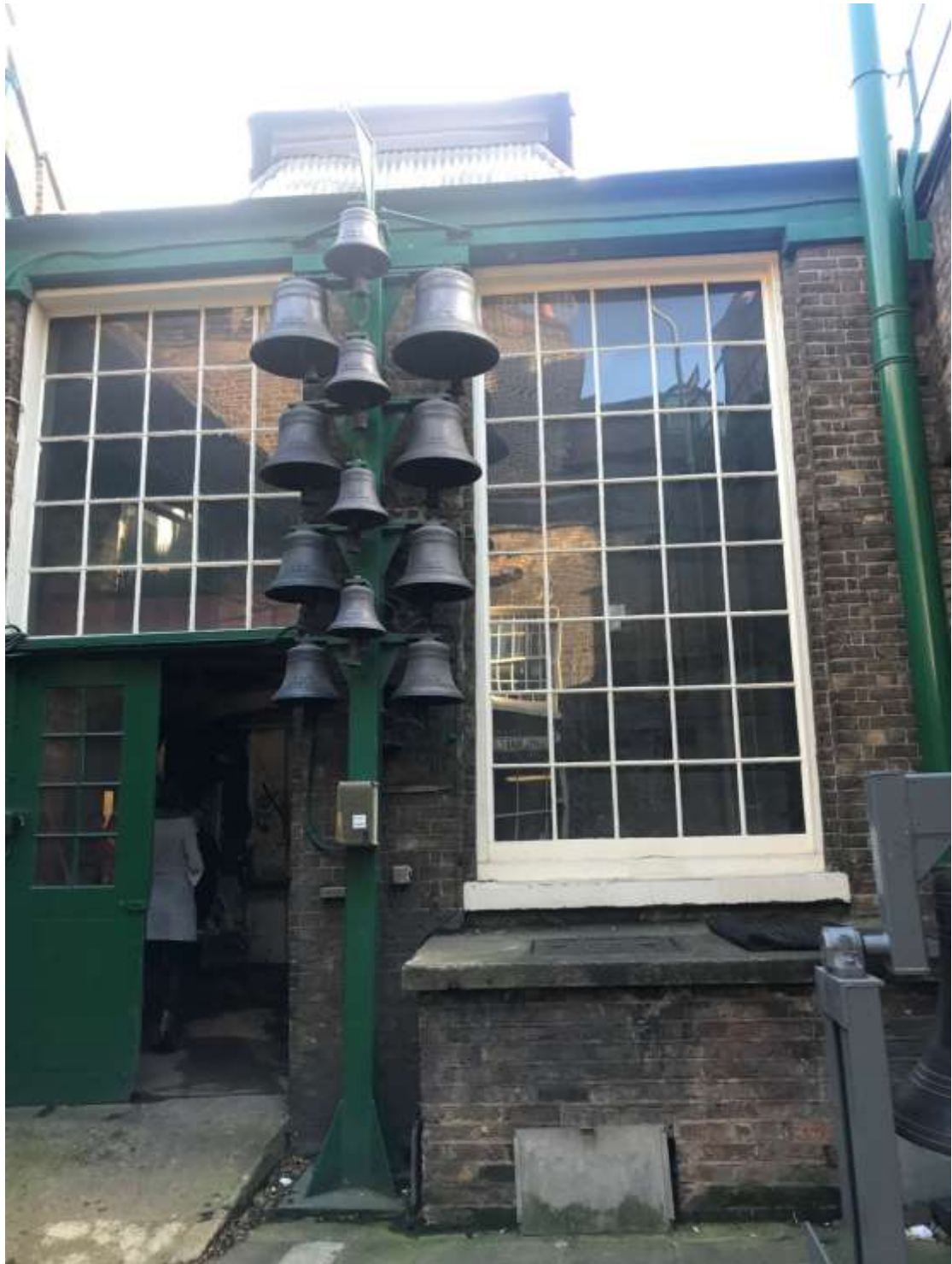
View on internal courtyard within foundry (facing south towards the 1980s extension and Mulberry Street)
