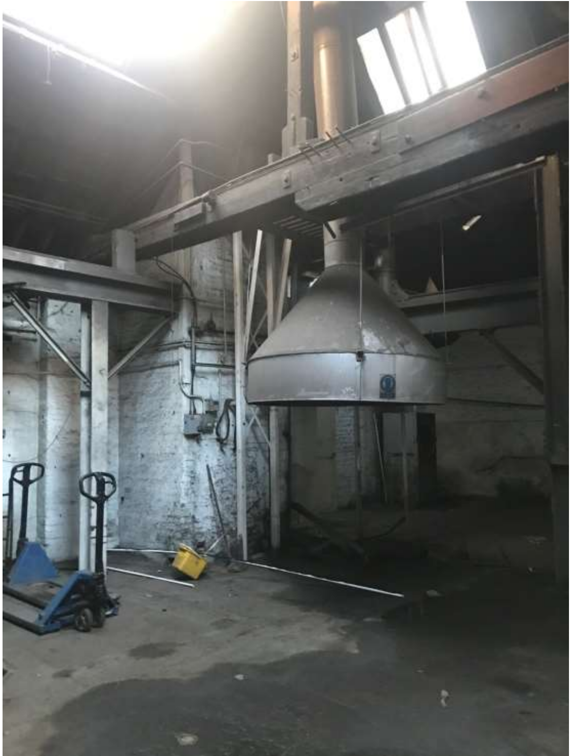
Existing space within historic foundry showing machinery that is part of the Grade II* listed fabric and to be retained
