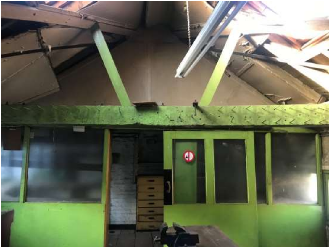
View from within upper workshops within Historic Foundry.
