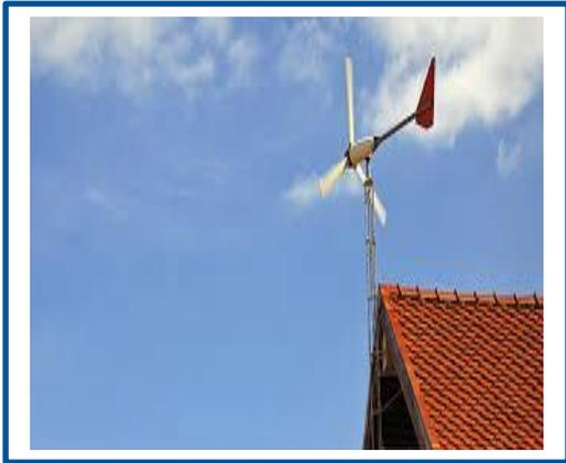
Typical wind turbines are rated between 650W and 2kW, with actual output generally well below this in normal wind conditions. The value of the electricity produced depends on whether it is substituting what the consumer would normally pay for mains electricity or whether it is exported and sold to an electricity company. Sites located adjacent to parks and open spaces and canals offer potential for small building mounted wind turbines.
