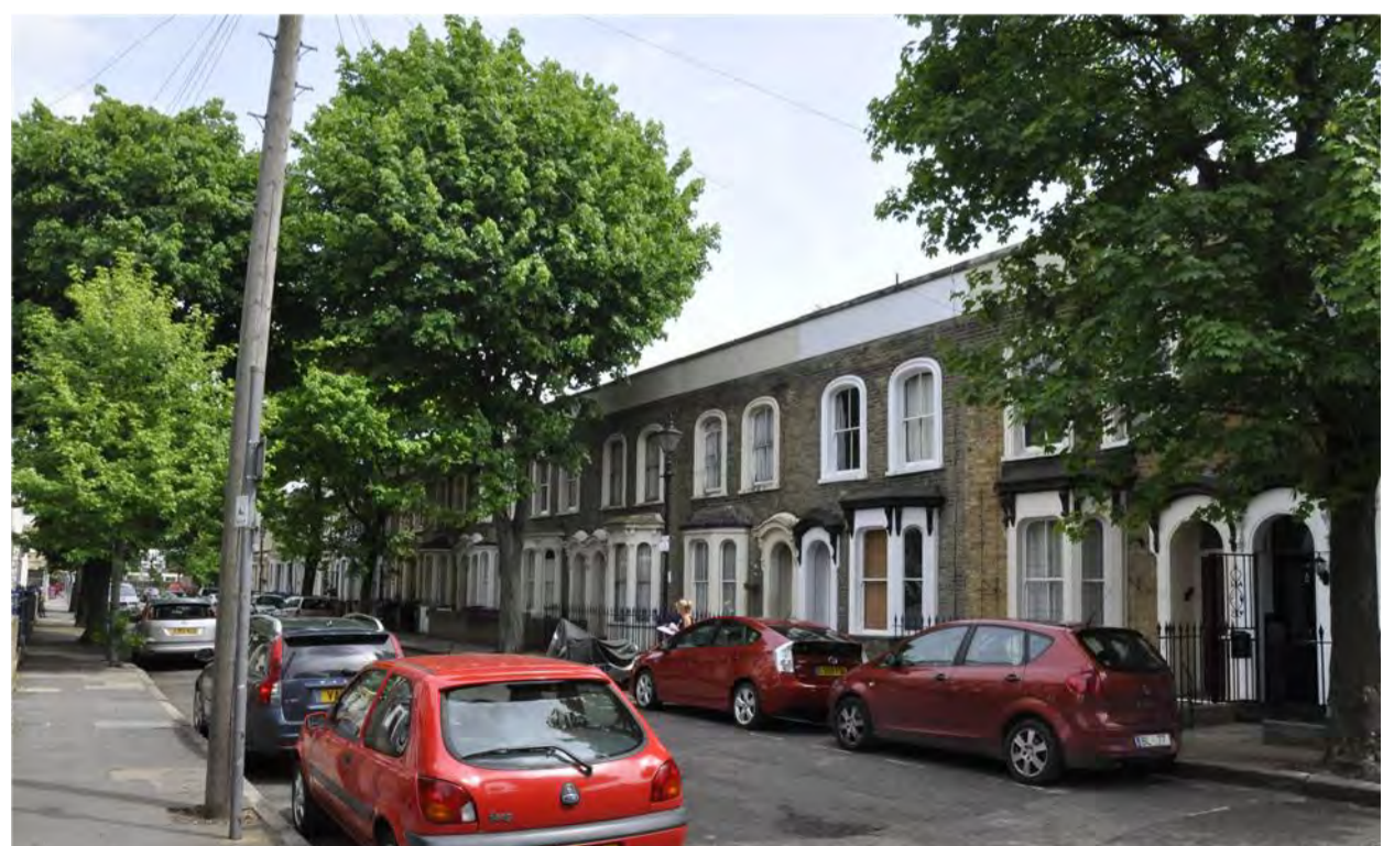
The same street in 2016 - the majority of cornices are missing
