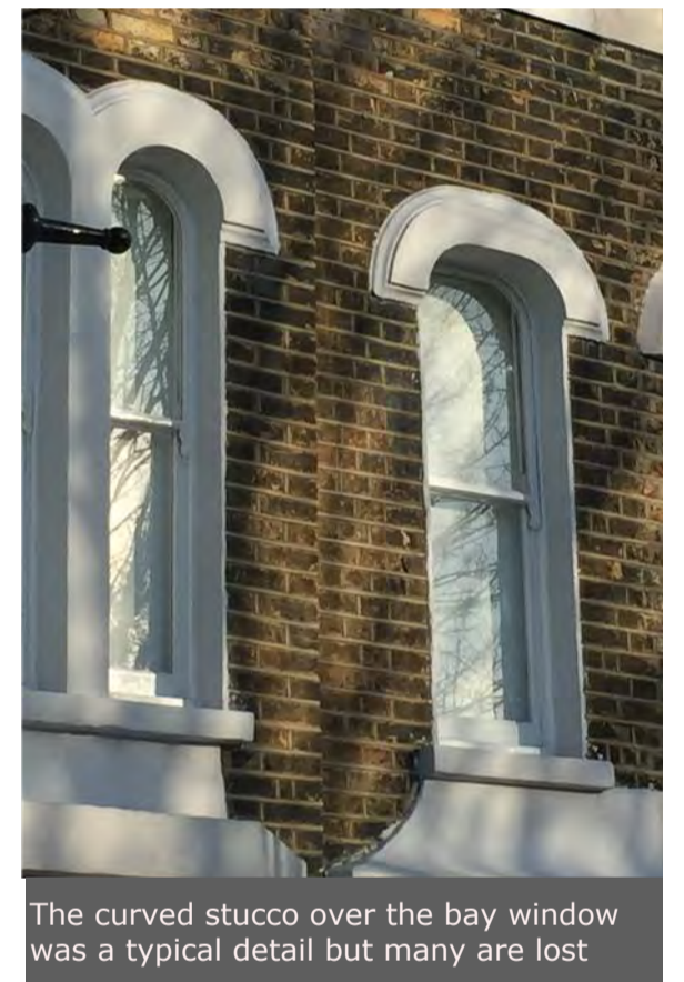
Typical curved stucco moulding over first floor windows in Medway Conservation Area
