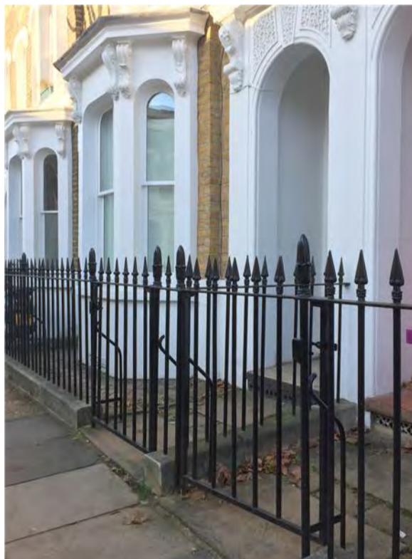
Antill Road replacement railings
