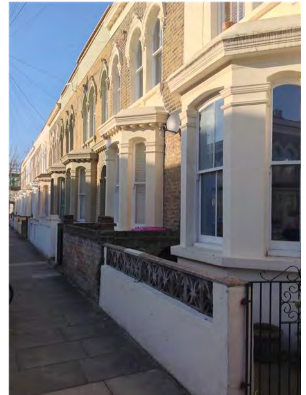
Strahan Road- loss of character
