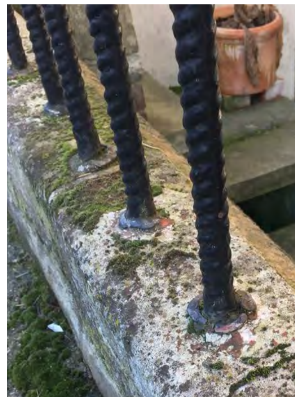
Bars lead caulked into stone base
