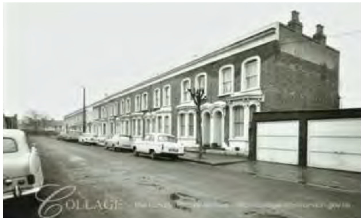
Post-war image shows the cornices intact Picture archive http://collage.cityoflondon.gov.uk/
