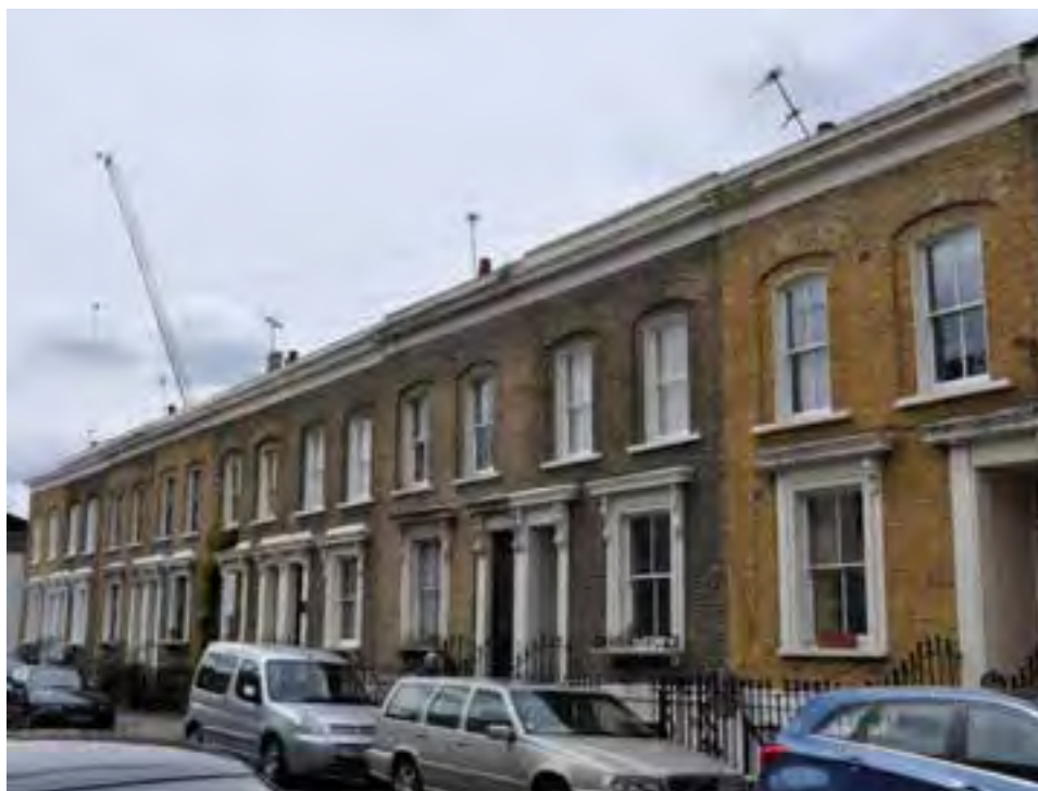
Two storey houses, with basements, along Ellesmere Road.
