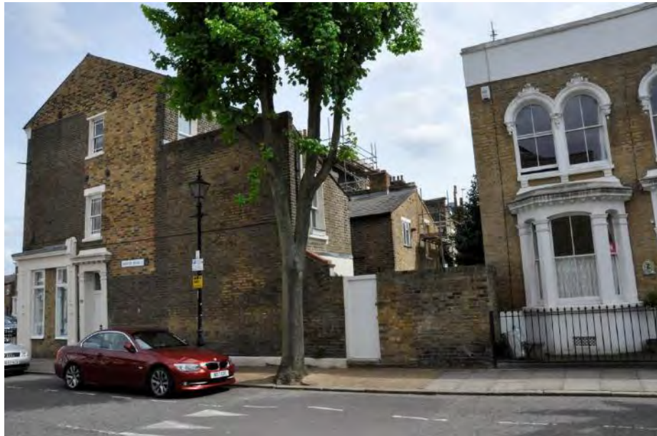
Rear extensions viewed from Arbery Road
