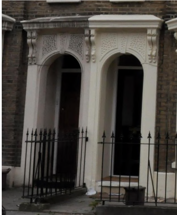
Detail showing reticulated rusticated stucco above the door.
