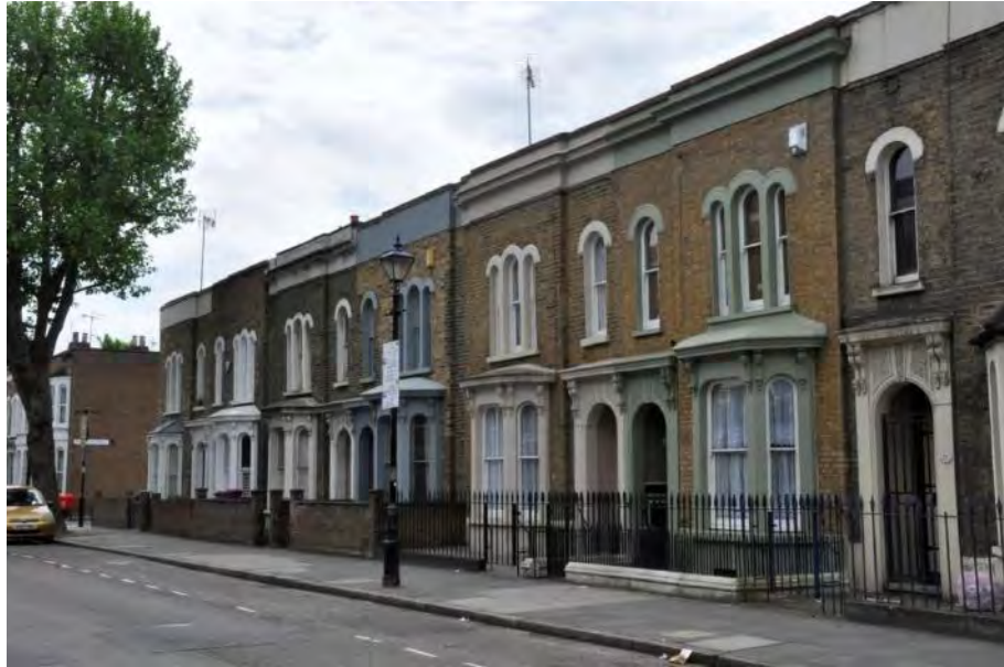
St Stephen's Road: note the tri-partite round-headed windows on the first floor, canted bay windows, and architectural embellishment to the door surround.
