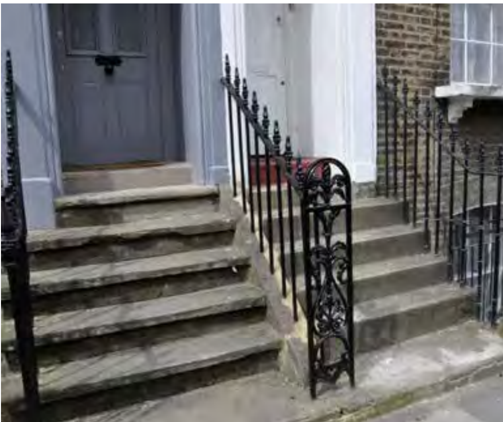
Below: Original wrought ironwork boot-scraper situated between two houses on Driffield Road. This design feature is also found on Grove Road. Also note, the loss of stone nosings to the modern steps on the right.
