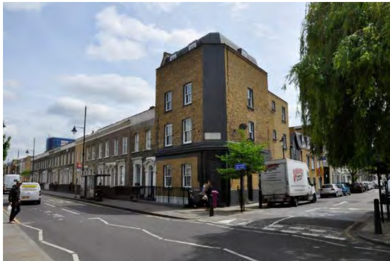
View of corner of Roman Road and Medway Road.
