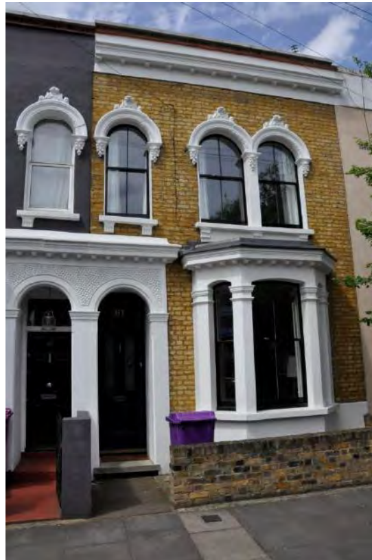
Strahan Road (with original cornice intact).
