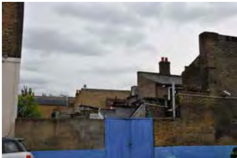
View from of Kenilworth Road: the rear elevations and closet wings of properties along Roman Road are visible.
