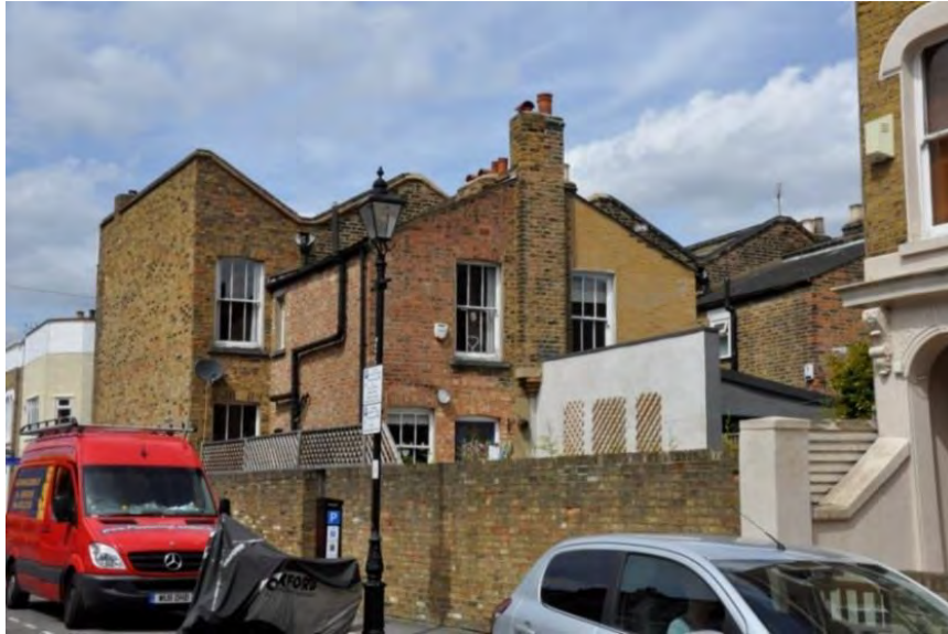
London Roofs visible along Medway Road.
