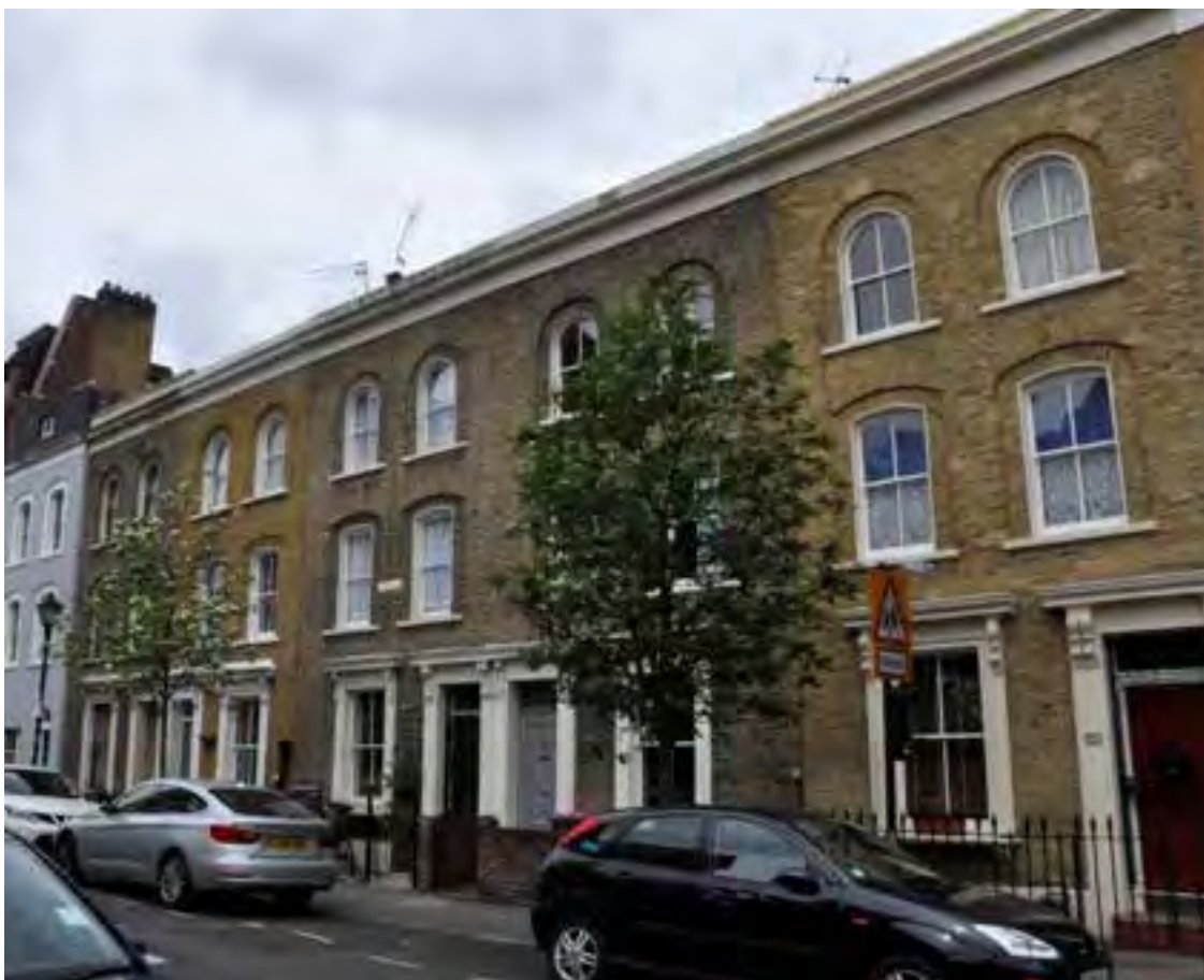
Chisenhale Road. Most houses have retained the original wrought iron railings but some (centre) have more recent brick walls to the front areas.
