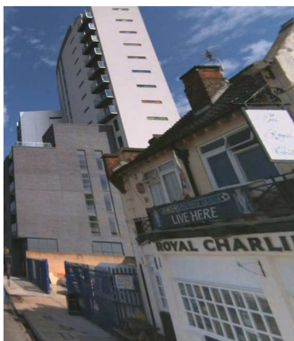
Photo 1: Parkview Apartments – Southern Elevation
