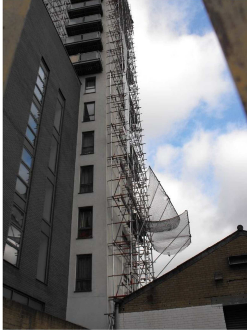
Photo 2: Part West Elevation - Parkview Apartments
