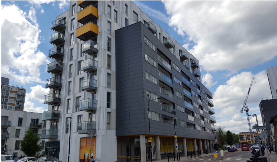
Photo 3: Equinox Building – Chrisp St Elevation
