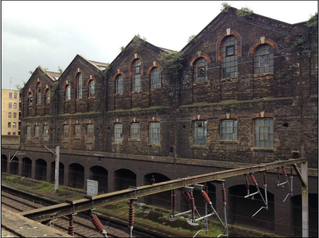
Figure 5: South-eastwards View of the Existing North Facade
