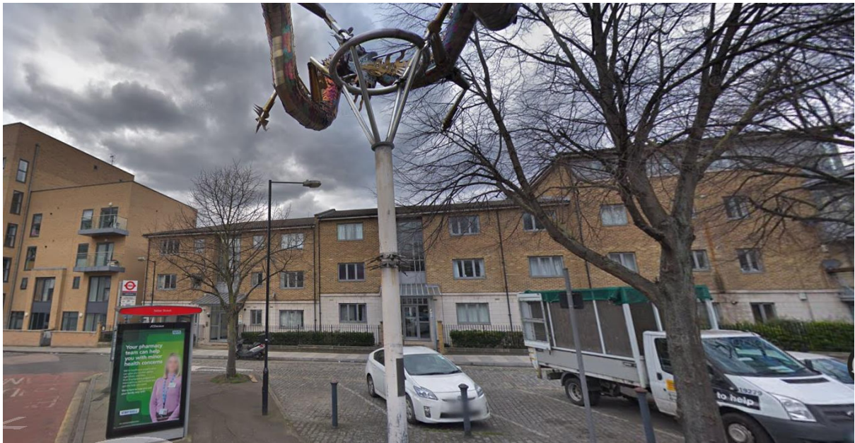
Eastern elevation of building from West India Dock Road
