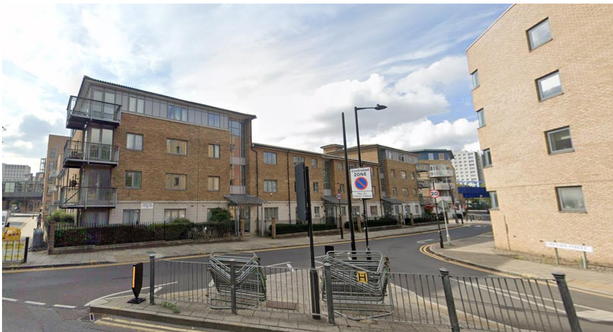
Northern elevation of building from West India Dock Road
