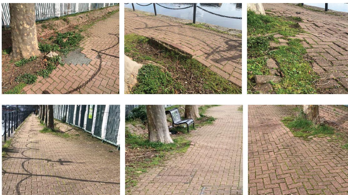
Figure 56: Photographs of existing towpath and conditions around trees
