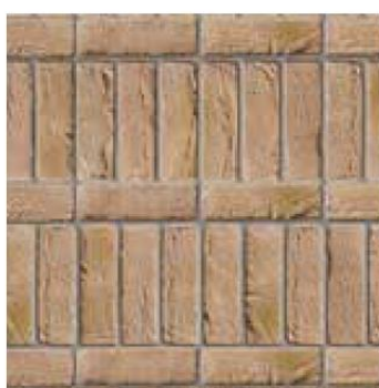
2. External Wall Detail (horizontal banding): Ibstock Brick-Bradgate (or similar) with Medium Grey Mortar
