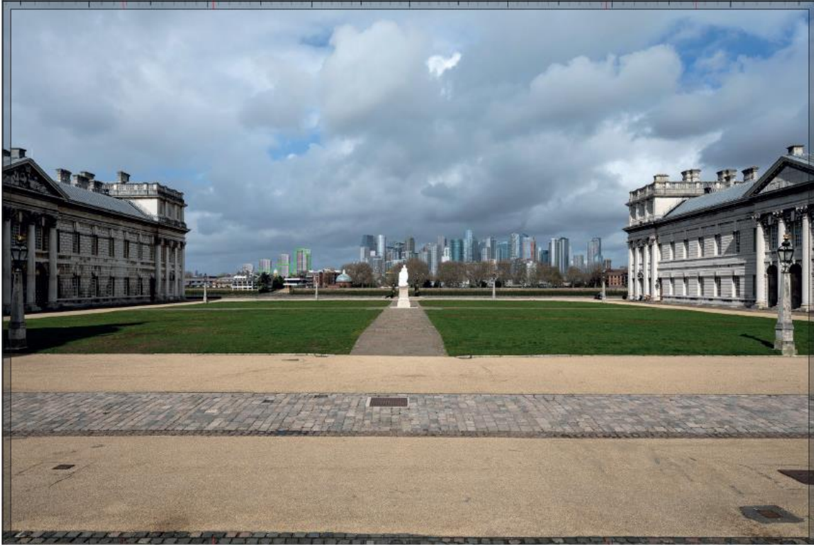
Figure 59: BHTVIA View 7 x 24 (Royal Naval College) cumulative View and consented scheme (green wire line)
