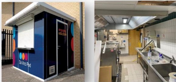
Images show a POD and on-going installation works to a kitchen.
